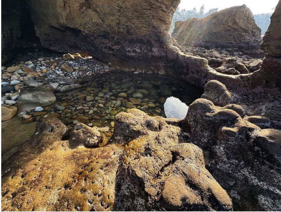
Figure 12b. Undercut and Eroded Section of Cliff, 2025. Located immediately upcoast of the Public Access Easement.
