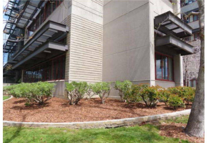
Image 5. Detail of scored concrete exterior walls, metal windows, and translucent awnings (ARG, 2024)
