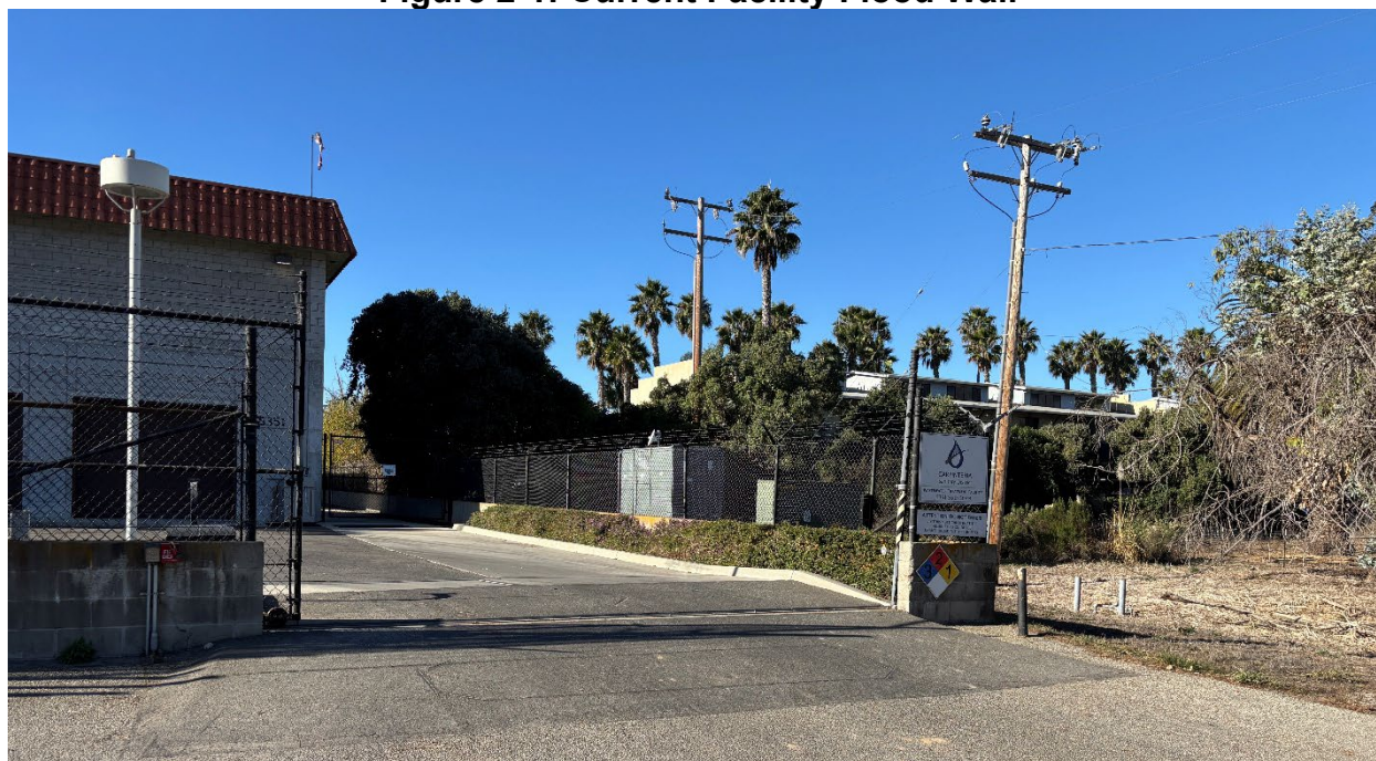
Figure 2-1: Current Facility Flood Wall
