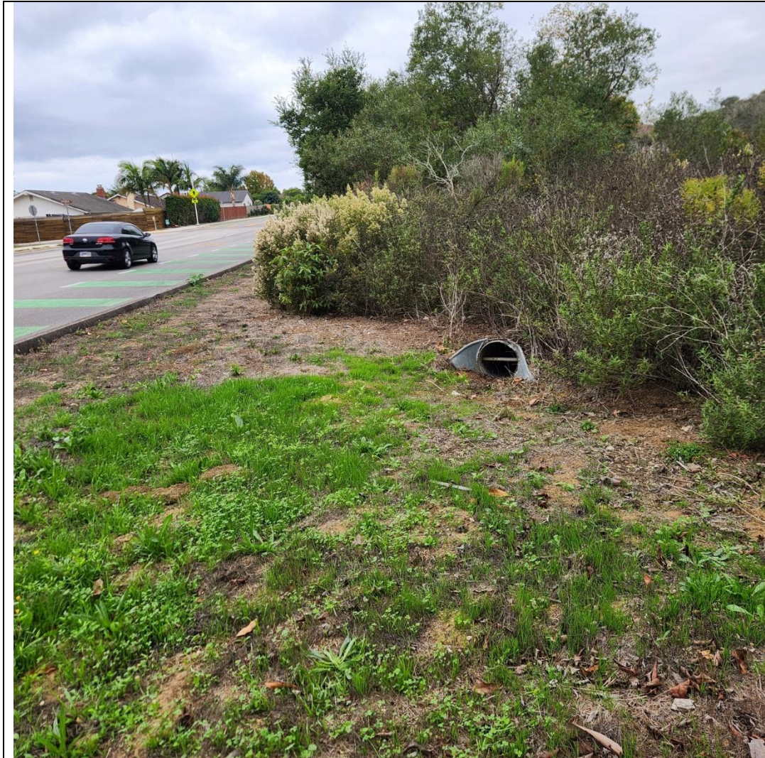
Photo 6. Existing storm drain culvert inlet adjacent to Cathedral Oaks Rd that outlets into El Encanto Creek. The new 90 ft. long storm drain from the new detention basin will tie into this storm drain. (view looking southwest taken, 11/5/2025)
