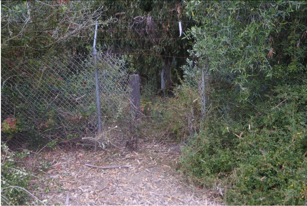
Photo 8. Gap cut in chain-link fence on the western property line of the Shelby 7400 Cathedral Oaks Rd property to provide access to El Encanto Creek (view looking west taken 7/11/2025)
