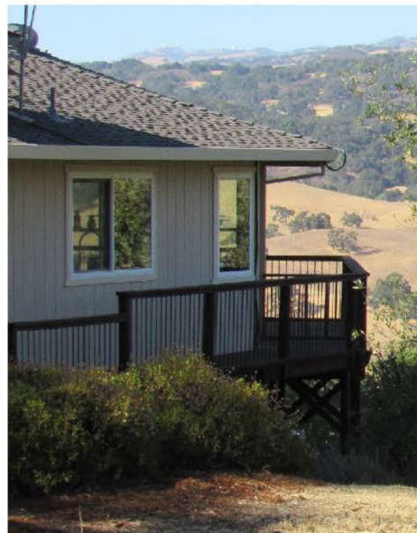
Photo 11. Elevated wood deck with direct exposure to hillside vegetation.
