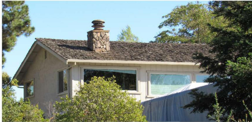
Photo 10. Weathered wood shingle roof. Siding is a mix of stucco and plywood.
