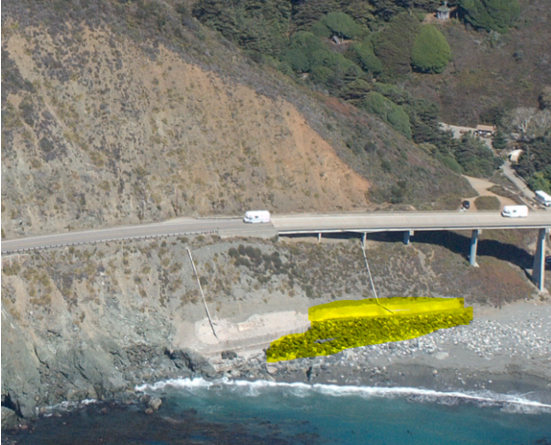
Figure 45 Revetment Removal
