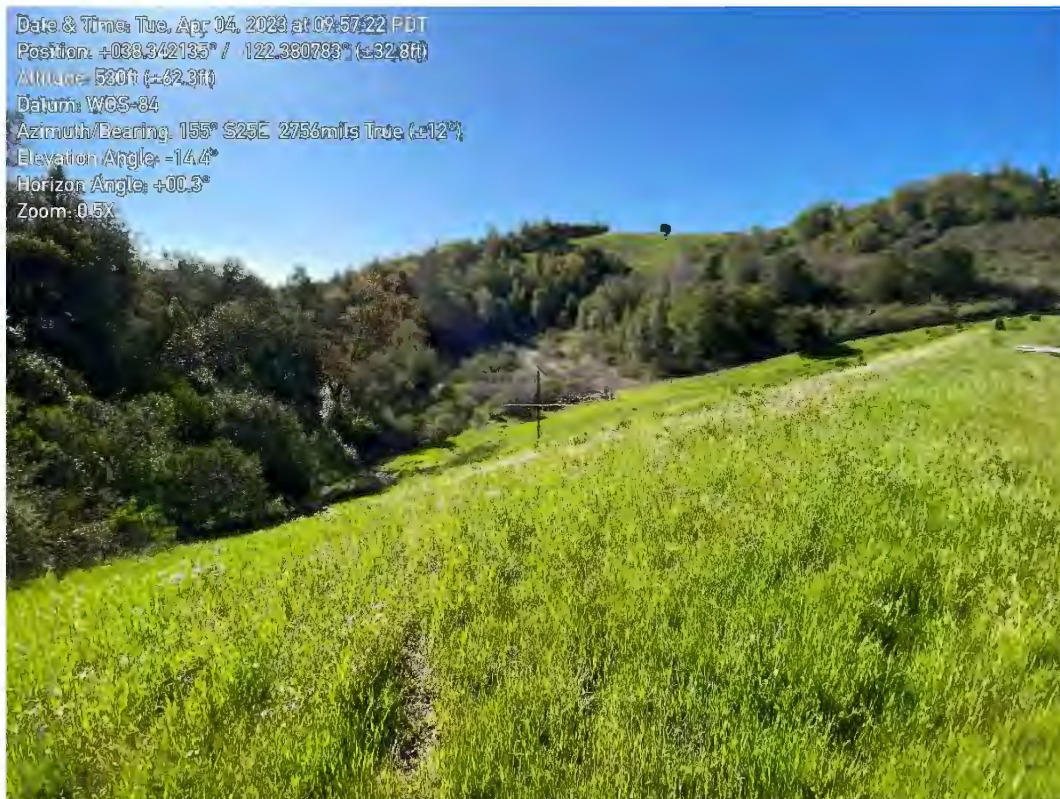
Photograph 5. Facing south at the face of the dam and hillside where construction will take place.
