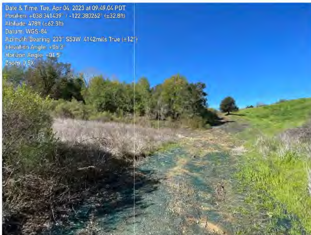
Photograph 6. Facing west upslope at the existing spillway and dam where construction will take place.
