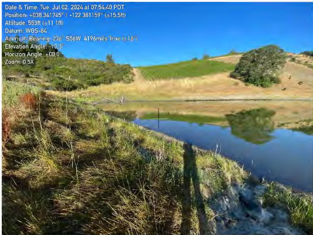
Photograph 7. Facing south across the water-side of the dam on 2 July 2024.
