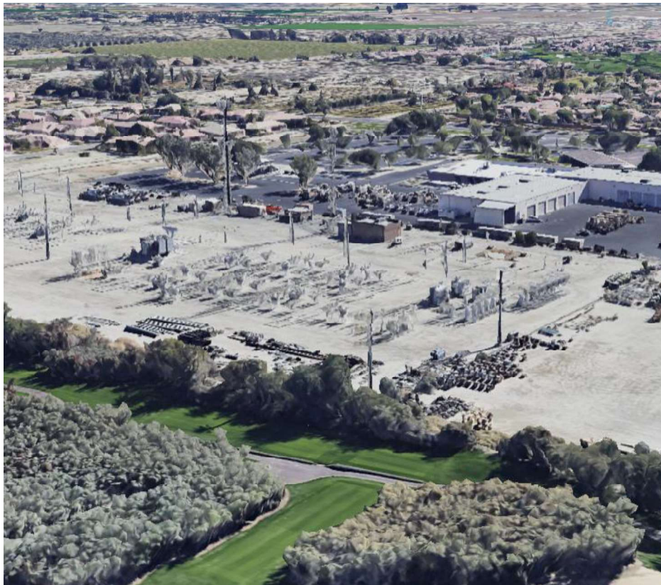
Photo 1: Aerial view of Avenue 58 Substation looking toward the southeast.
