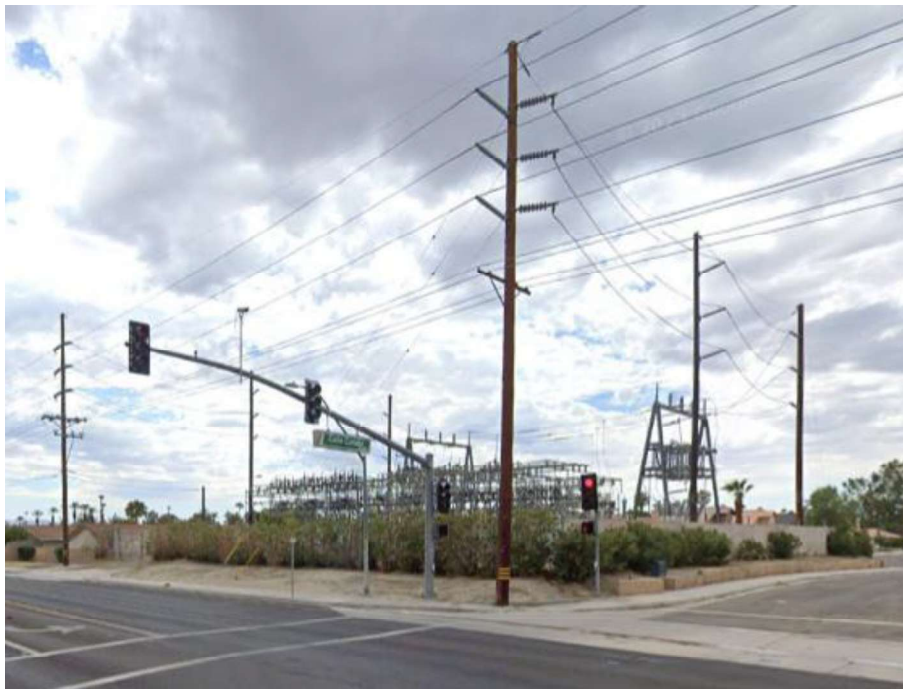
Photo 3: View of example line section for replacement of 92kV single circuit (Hjorth Street).
