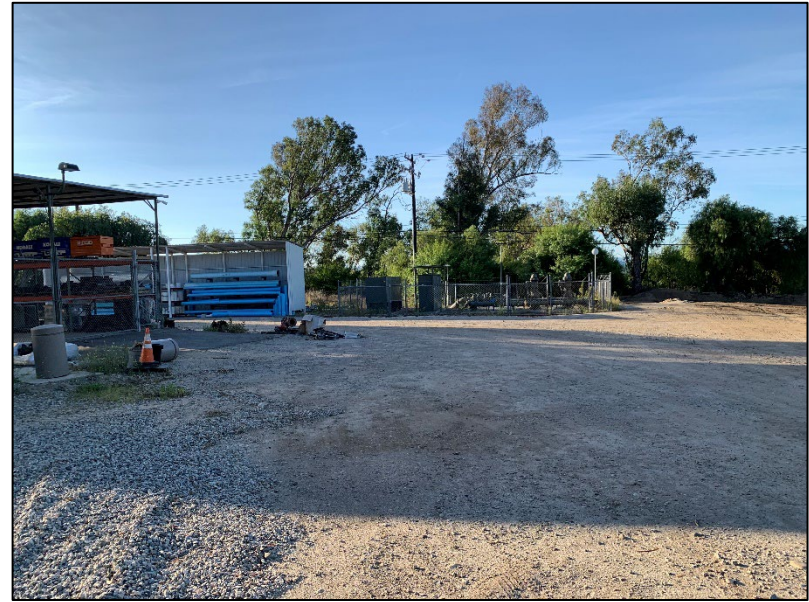
b. Existing storage facilities and booster pump station (background)
