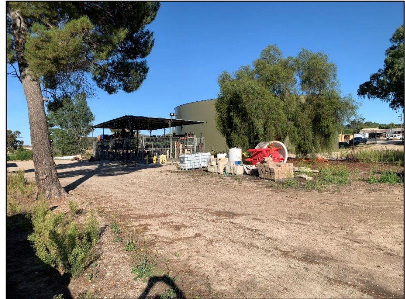
d. Existing tank and storage shed, facing west
