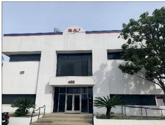
Office and Administration Building
