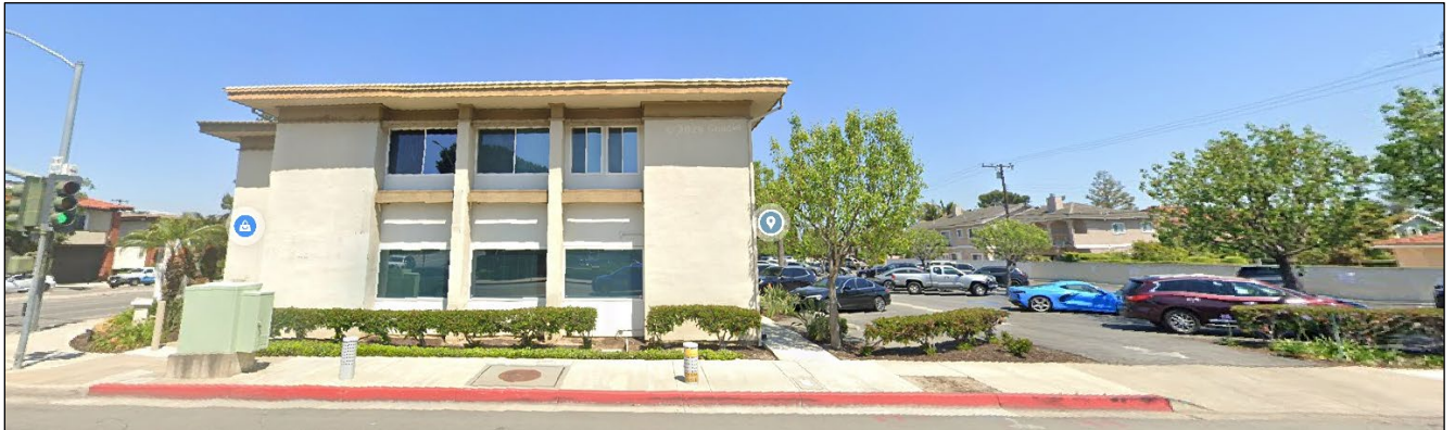
Figure 4. Photo of Existing Building, East Elevation From Yorba Street
