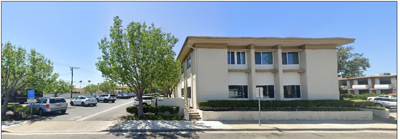
Figure 5. Photo of Existing Building, West Elevation From Mountain View Drive
