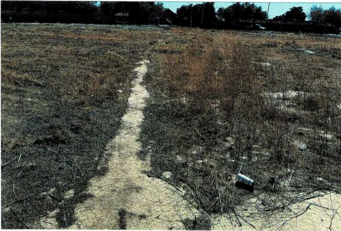
Photo #7: An excavated strip runs SE to NW for 100 ft. from where the former farm buildings were located. It appears the former septic tank, overflow basin and the sewer line have been removed.
