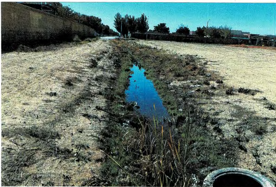
Photo #6: A storm water drainage ditch runs along 27 th St. East. Note 27 th St. is unfinished.
