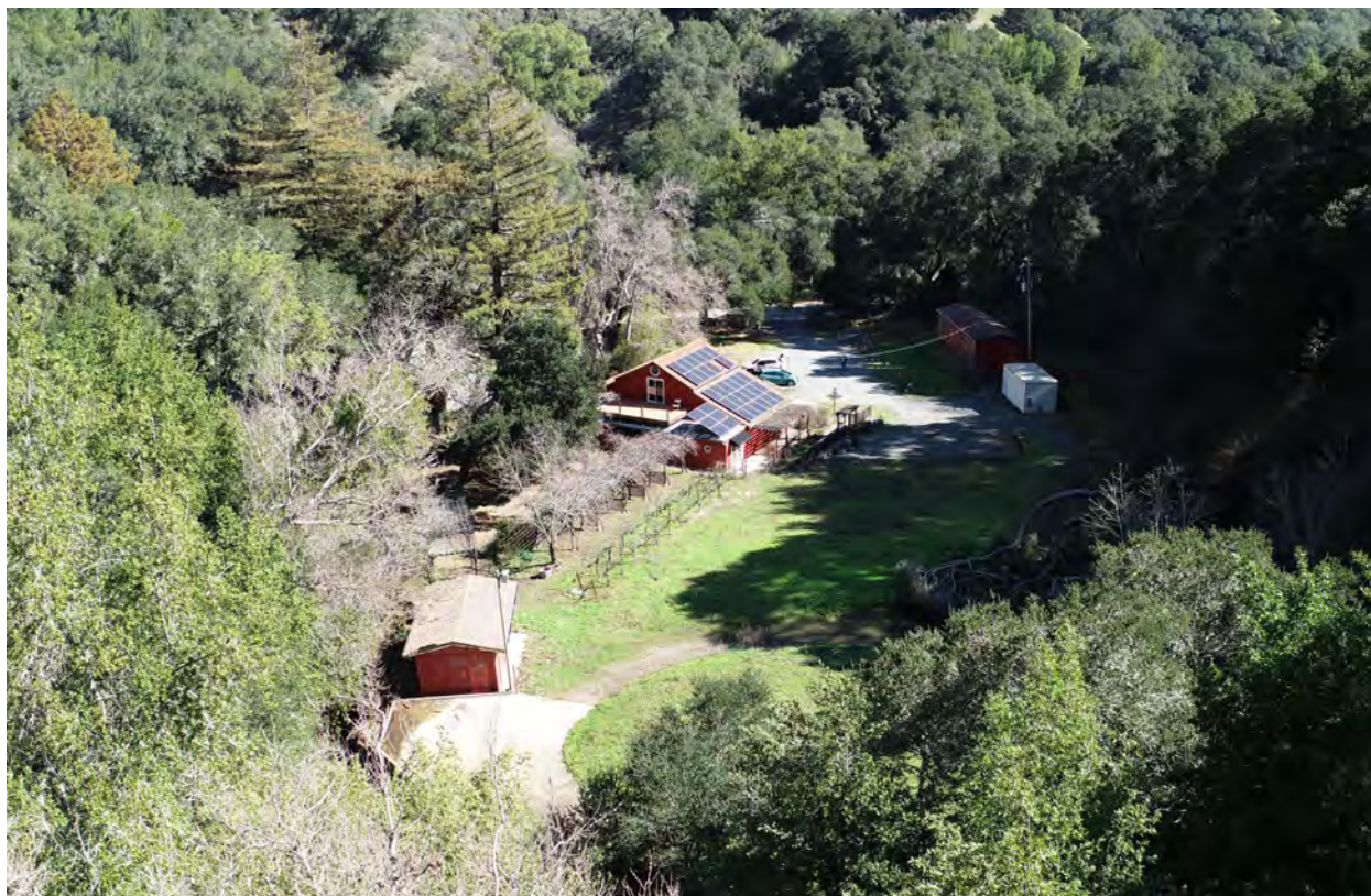
Figure 3 Existing Photo of Chouinard Property Looking East
