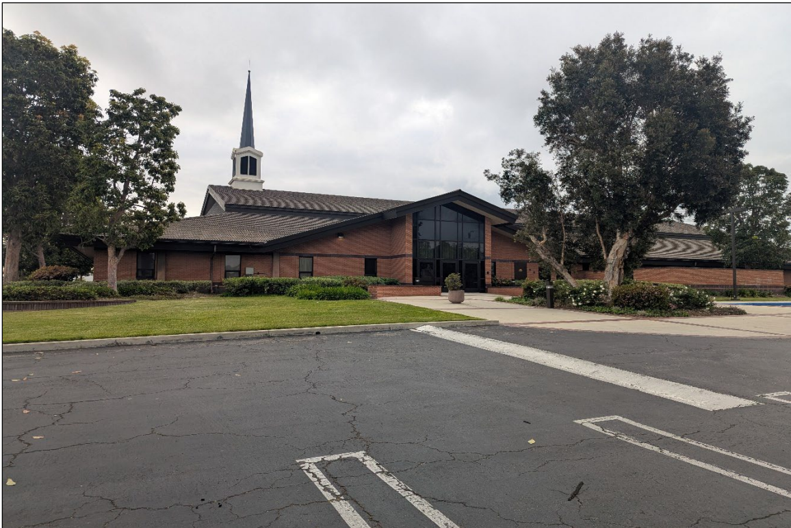
Figure 4-3 Overview of 2000 Artesia Boulevard, facing northeast.
