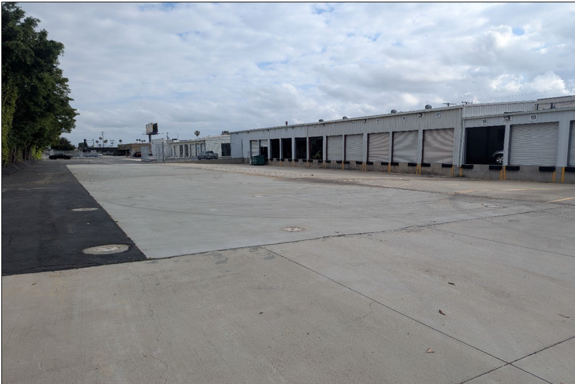
Figure 4-5 Overview of 1942 Artesia Boulevard, facing northeast.
