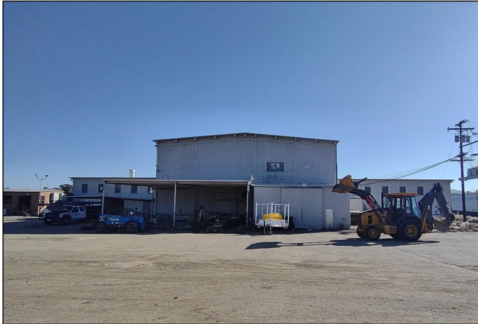
Plate 6. North elevation, facing south.
