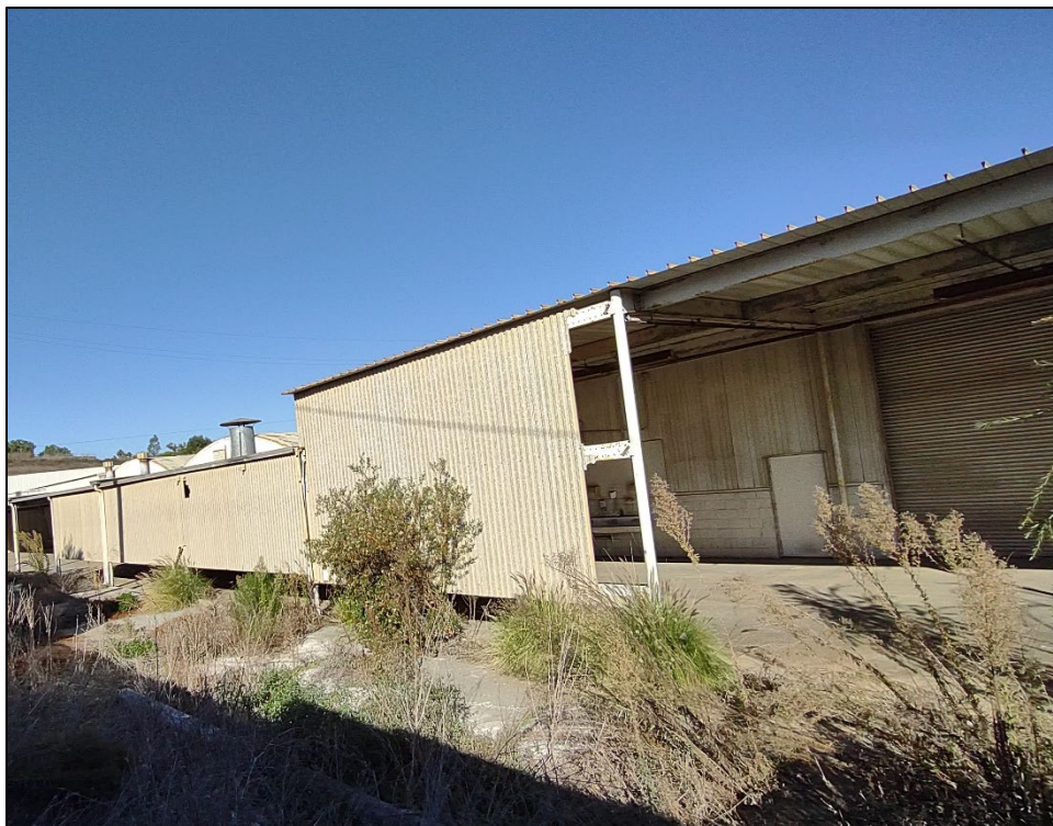
Plate 13. West Building east elevation central section, facing northeast.
