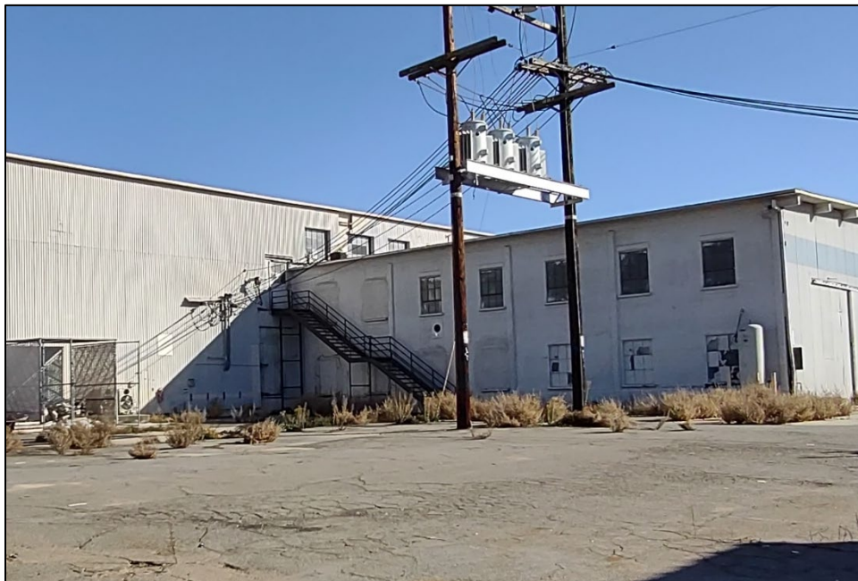
Plate 7. North elevation, west bay, facing southeast.
