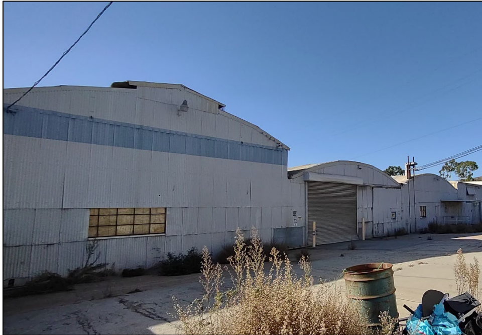
Plate 17. West Building east elevation central Quonset-roofed section, facing northwest.
