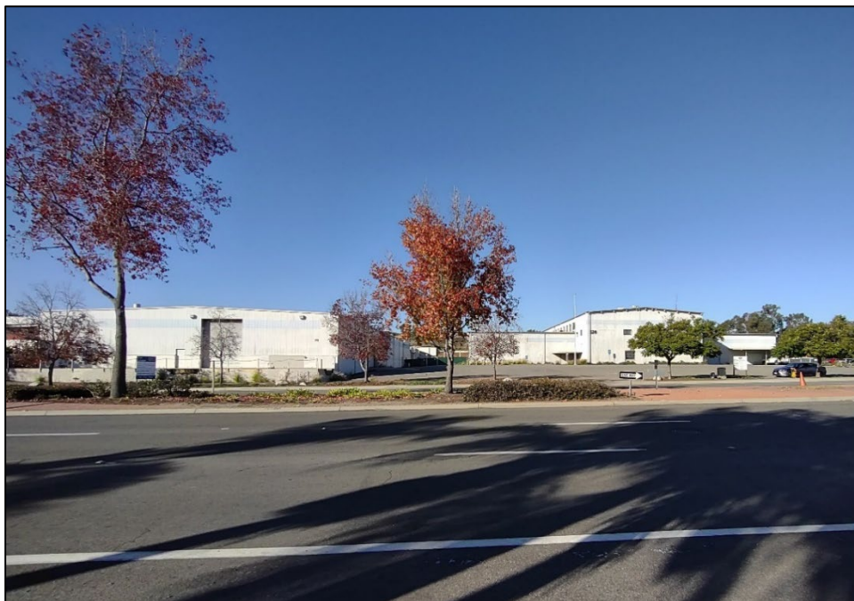
Plate 2. 528 East Mission Road, facing north.
