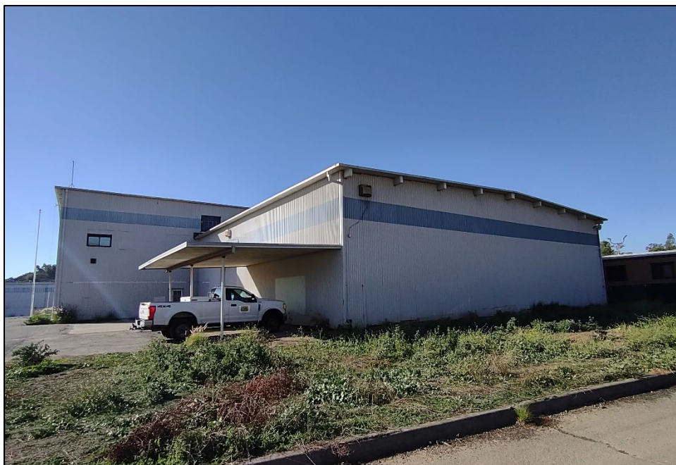
Plate 10. East elevation south end, facing northwest.
