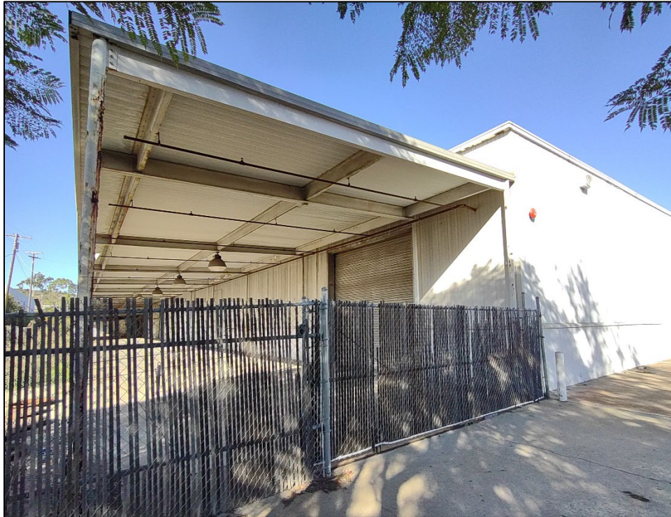
Plate 12. West Building east elevation, southwest corner, facing northeast.
