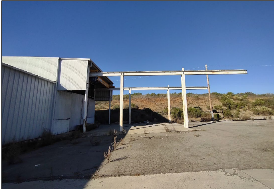
Plate 16. West Building north/south elevation crane hoist (as viewed from the south, facing north).
