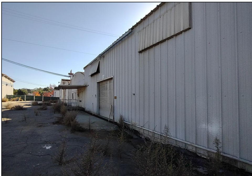
Plate 18. West Building east elevation northerly section showing wide ribbed siding, roll-up door, and covered upper windows, facing south.
