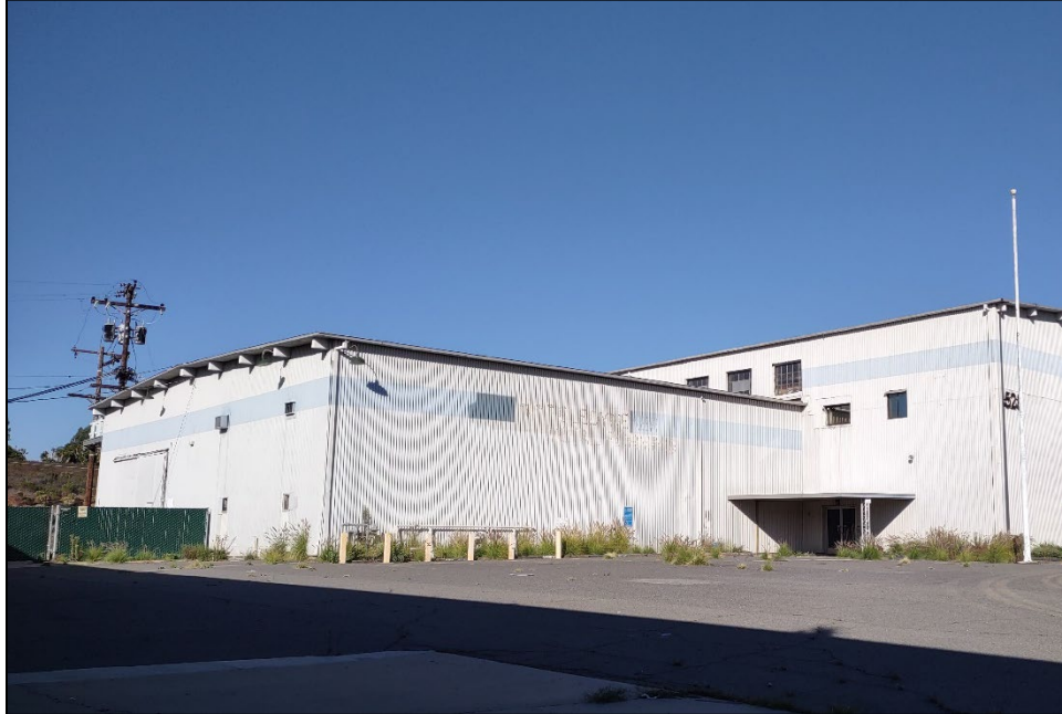
Plate 4. West elevation south end, facing northeast.
