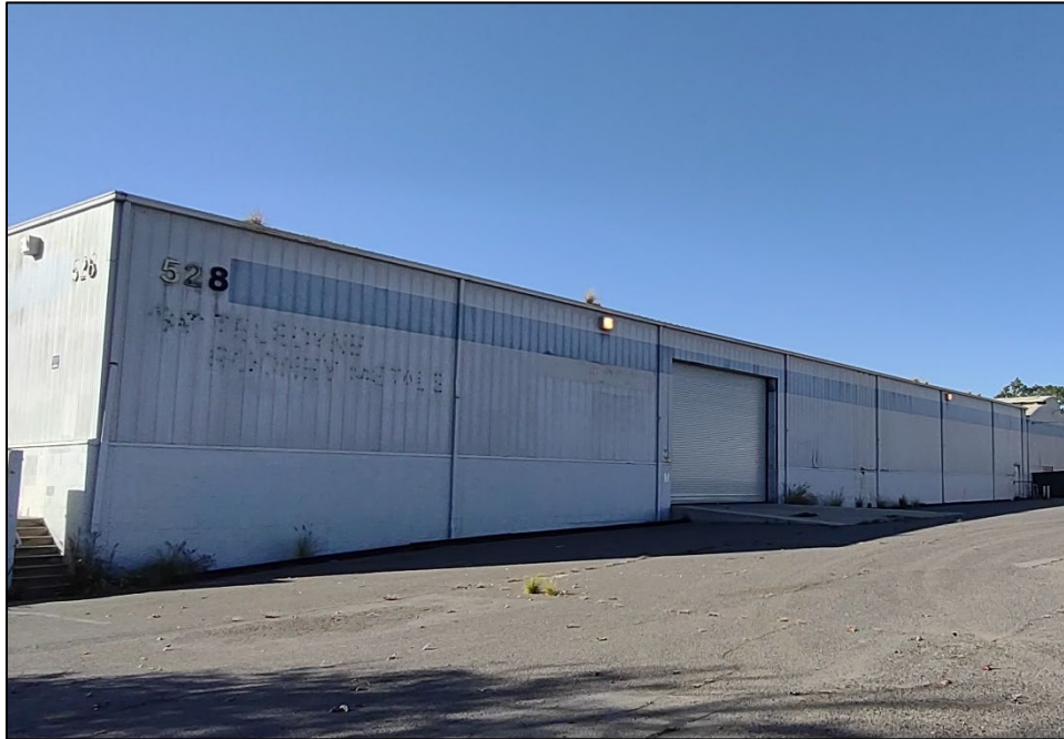
Plate 19. West Building east elevation southerly section, facing northwest.
