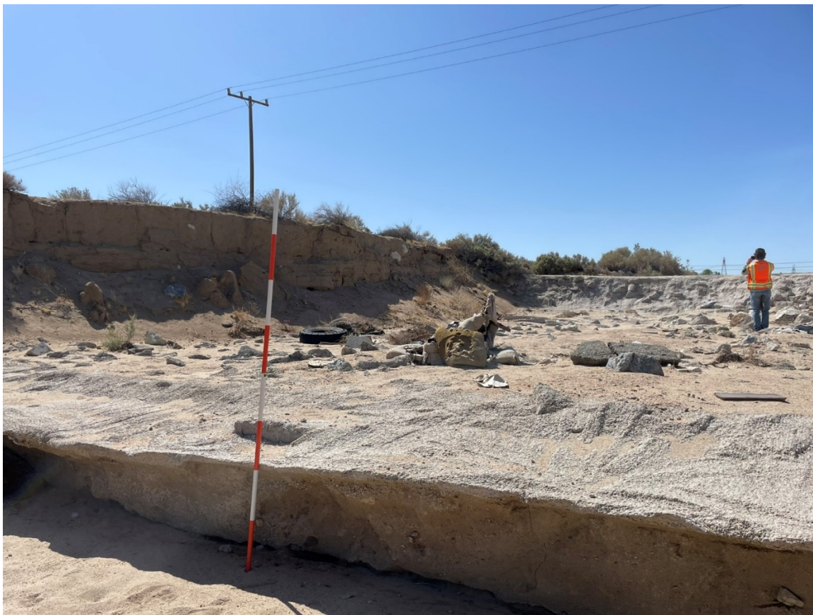
Figure 3.1: Existing Conditions Grouted Rock Channel
