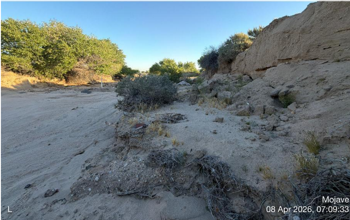
Photo 3. View of eroded western bank
