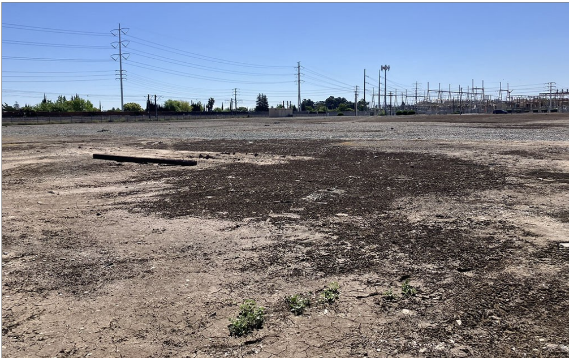
Source: Photograph taken by Ascent in 2026. Barren land cover at new Meadowview Substation site.
