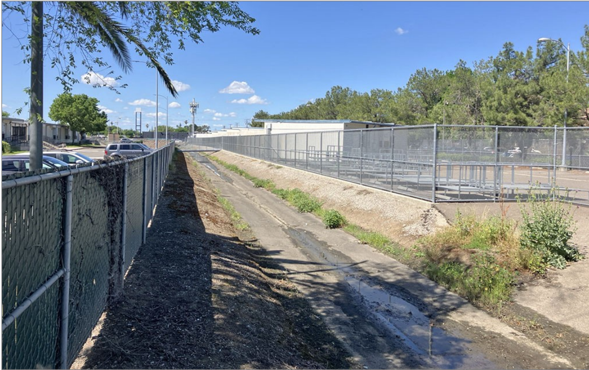
Source: Photograph taken by Ascent in 2026. Riverine drainage beneath 25th Street.
