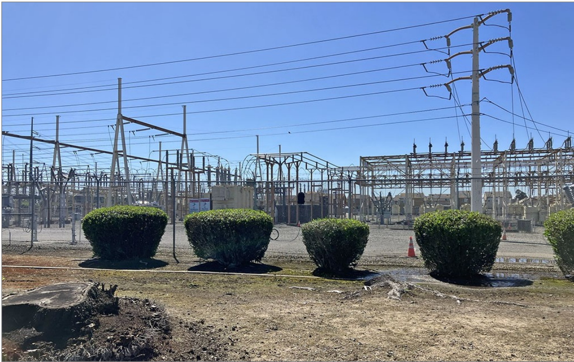
Source: Photograph taken by Ascent in 2026. Existing Pocket Substation site and ornamental shrubs.
