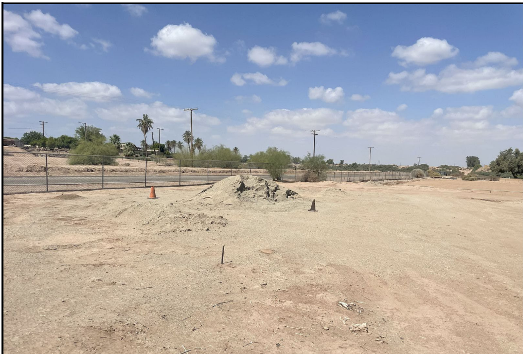
PHOTOGRAPH 6 Stockpile of Import Material along Southern APE Boundary; Looking Southwest
