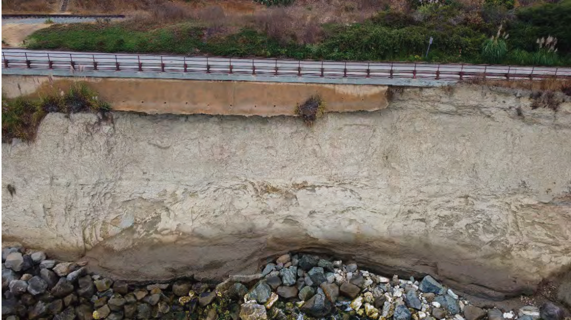
Photo 2: View of existing nail wall with eroding bluff below
