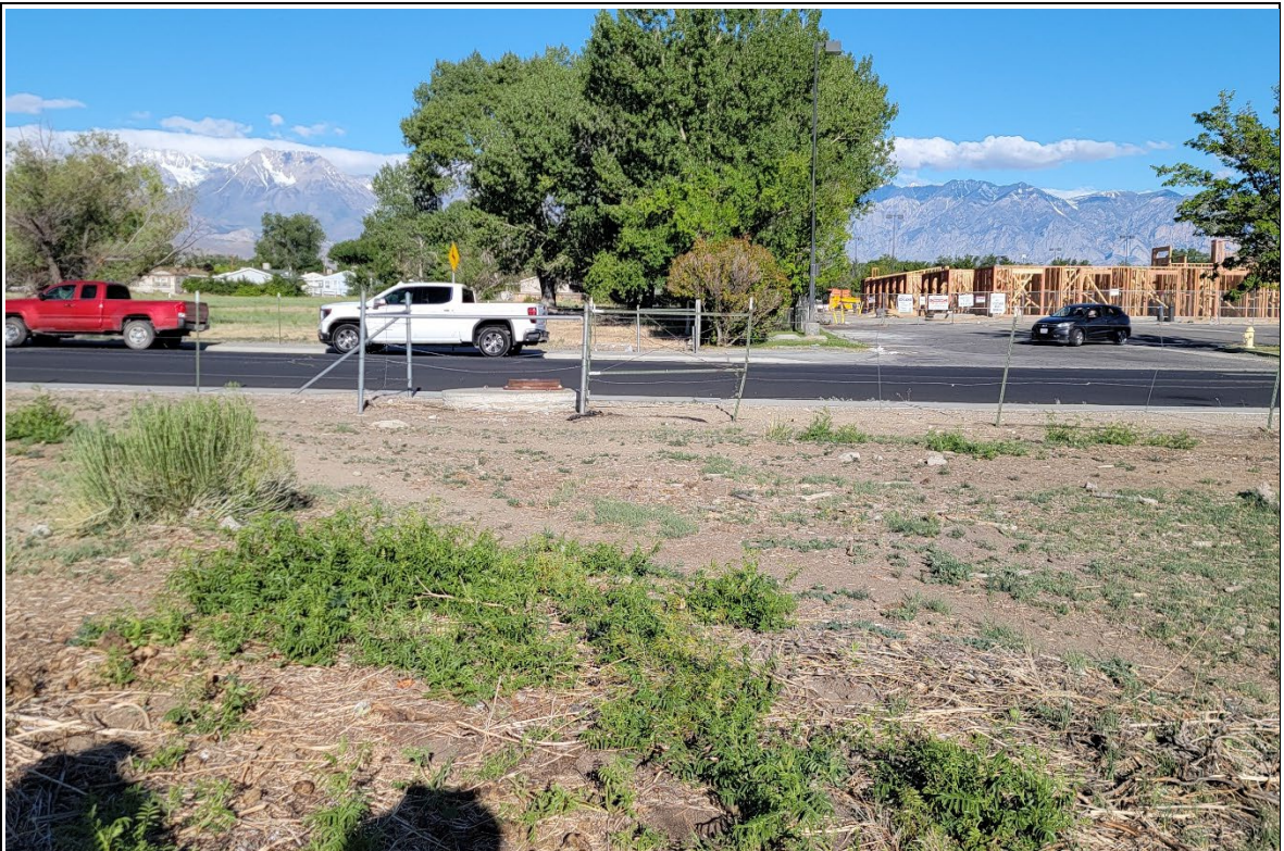
Photograph 1: Photograph depicts western most manhole situated along ESCSD Collection System Segment between Spruce Street and East Yaney Street, facing west (Taken on 05/27/2026).
