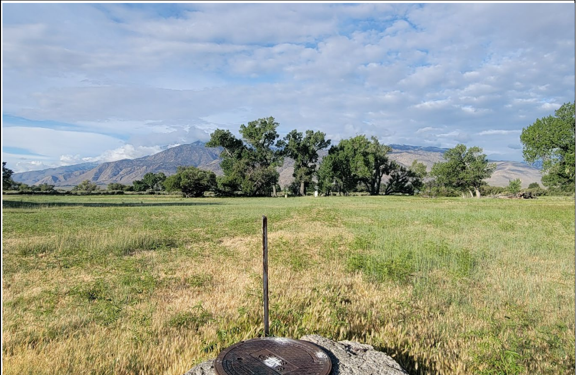
Photograph 6: Photograph depicts ESCSD Collection System Segment east of U.S. Route 395 and south of East South Road, facing southeast (Taken on 05/28/2026).
