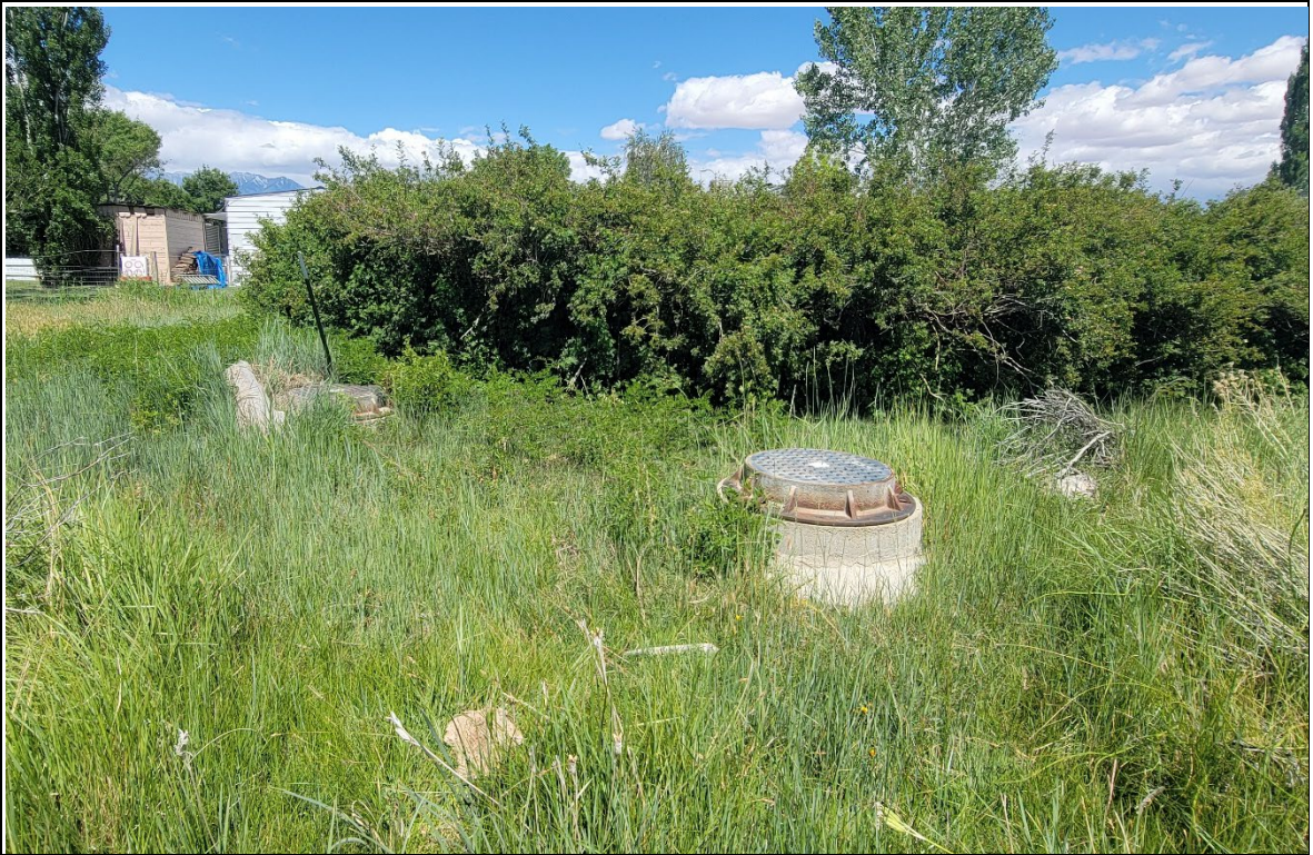
Photograph 5: Photograph depicts ESCSD Collection System Segment northeast of U.S. Route 395 and U.S. Route 6 where segment intersects the Highlands Family Mobile Home Community, facing northwest (Taken on 05/27/2026).
