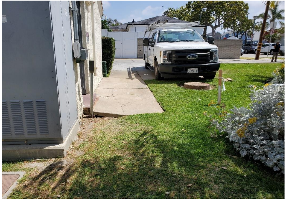
Photograph 1: Southeast side of S-7 sewer lift station, looking northeast.
