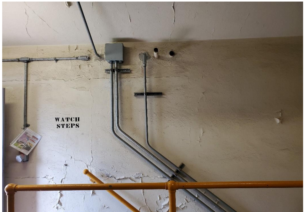
Photograph 16: Continuation of crack in photograph 15, on the southwest wall.
