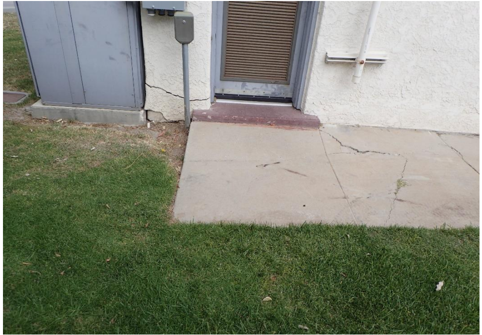
Photograph 3: Southeast side of S-7 sewer lift station, looking northwest.
