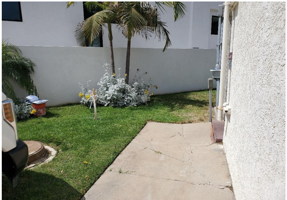
Photograph 2: Southeast side of S-7 sewer lift station, looking southwest.
