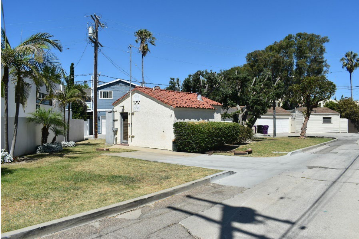
Figure 10. Overview of Sewer Lift Station S-7 Parcel, Viewing West.
