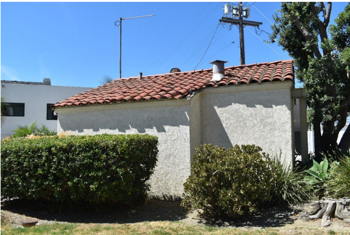
Figure 15. Superstructure, East Elevation, Viewing Southwest
