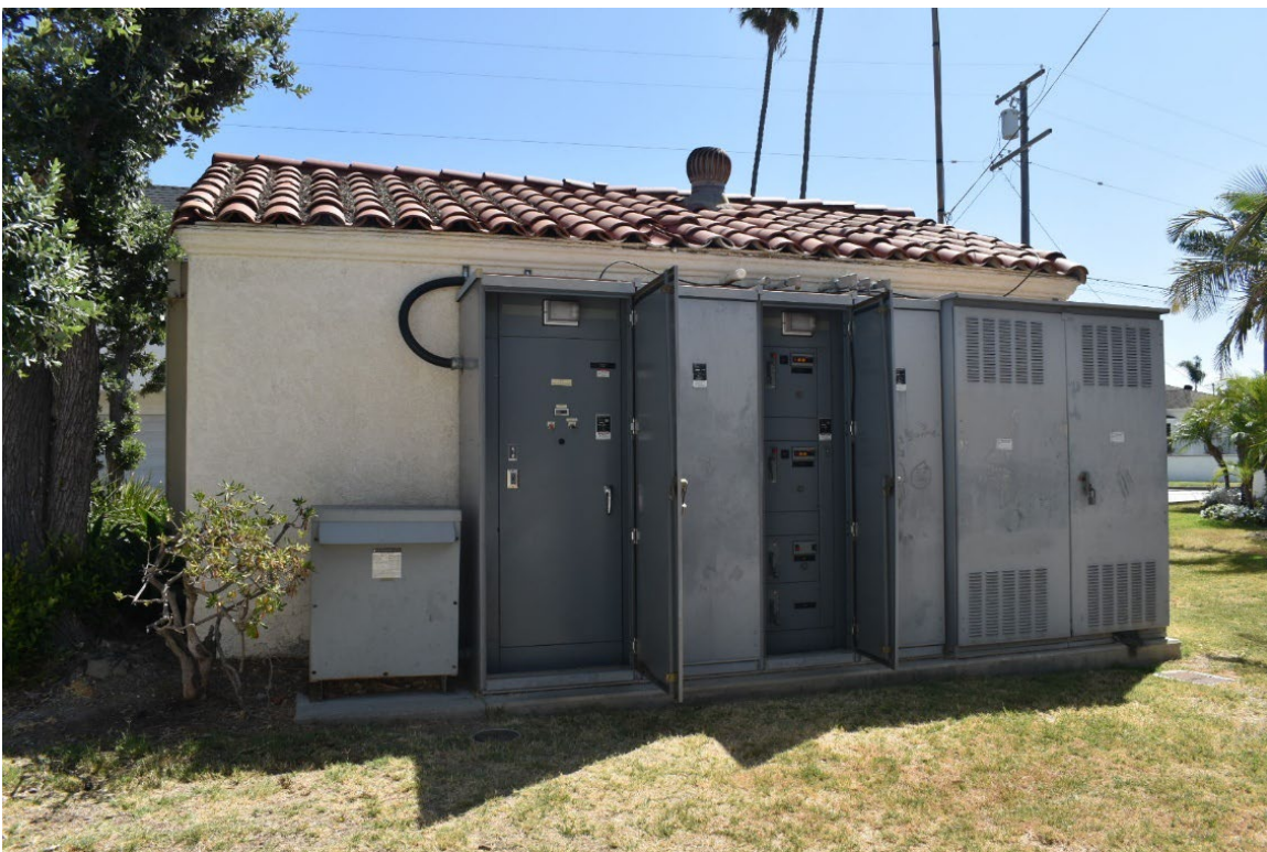
Figure 13. Superstructure, West Elevation, Viewing East
