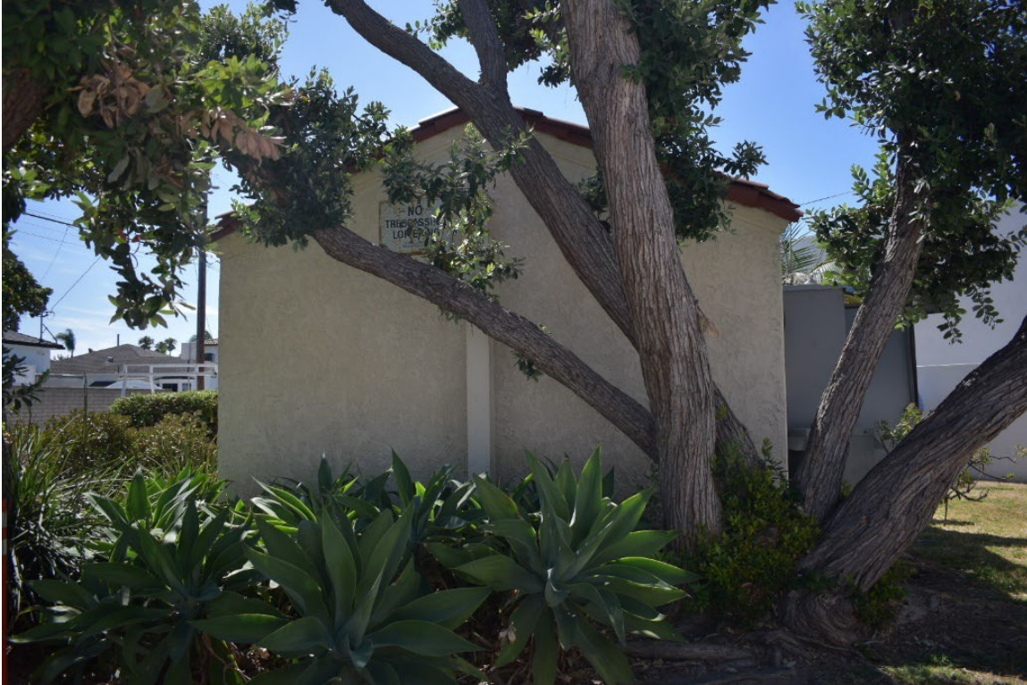
Figure 14. Superstructure, Rear (North Elevation), Viewing Southeast
