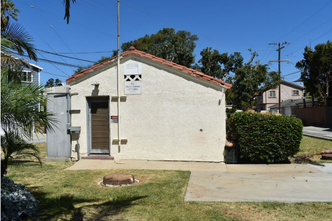
Figure 12. Superstructure, Façade (South Elevation), Viewing North
