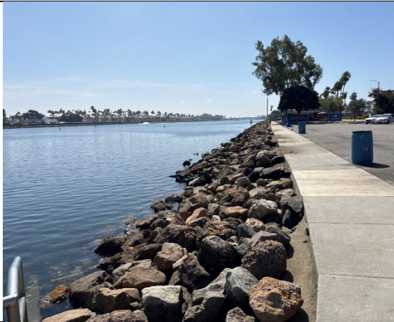
Photograph 7. View looking southeast along Marine Stadium riprap at the edge of Will Rogers Mini Park.
