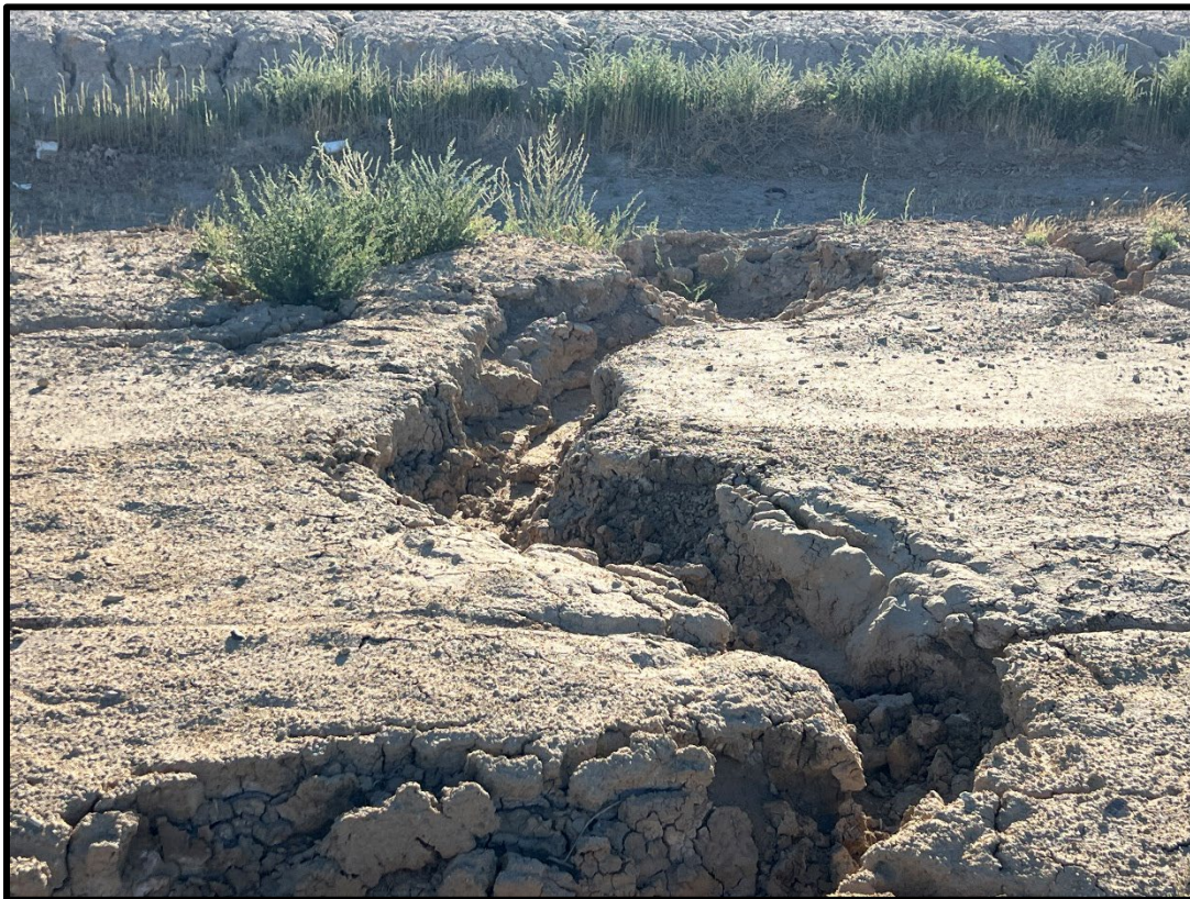
Top photo depicts the drainage along western boundary. Largest erosional feature shown in bottom photo. This feature was approximately 10 feet long and situated within the western graded area which consists of soft clay loam.
