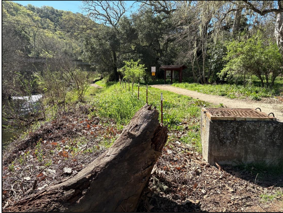
Photo 5. View south of intake structure above top of bank of Atascadero Creek (03-02-2026).
