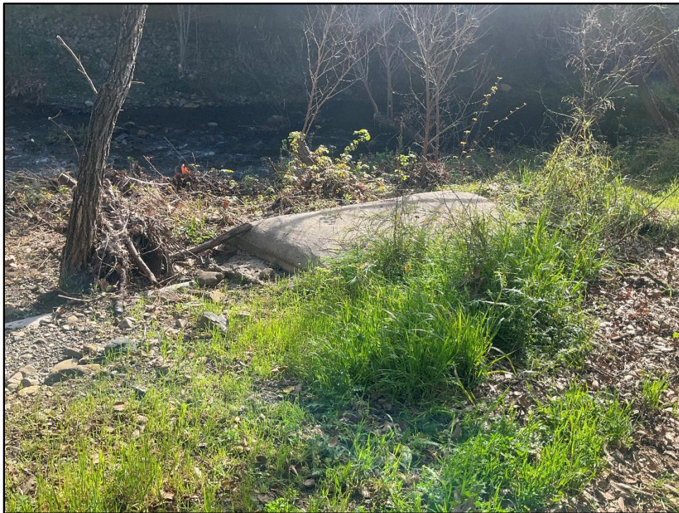
Photo 2. View east of concrete hold-down on banks of Atascadero Creek (03-02-2026).
