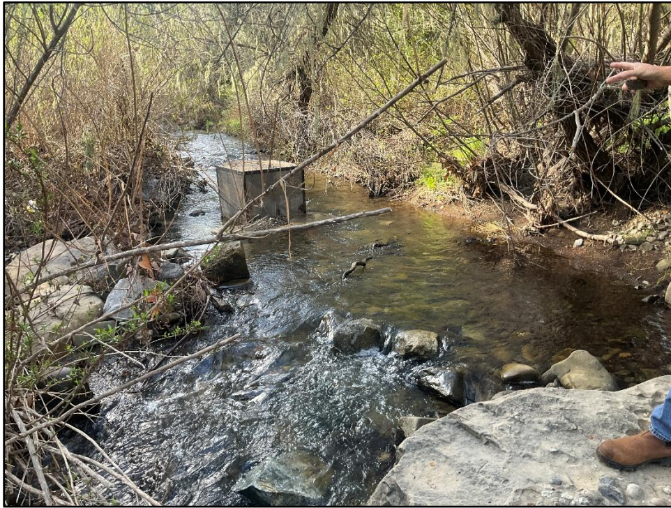
Photo 1. View south of intake structure in Atascadero Creek (03-02-2026).
