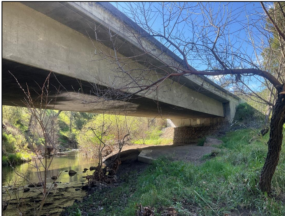
Photo 4. View south of project area below CA Highway 41 bridge (03-02-2026).
