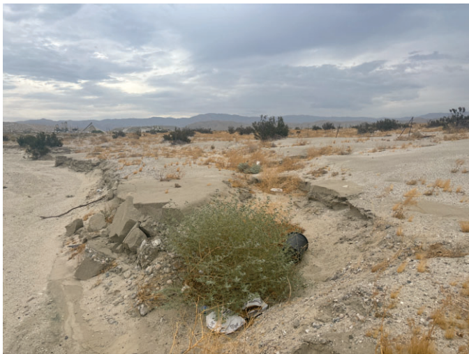
Photo 5: View looking northeast where Drainage 1C flows southwest into Drainage 1.
