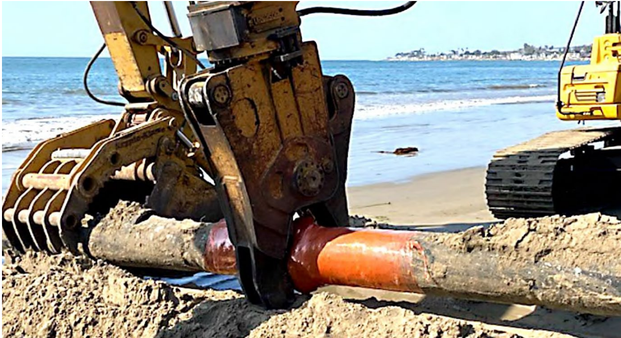
Figure 2-4. Photograph of Pipeline Cutting with Excavator-Mounted Shear
