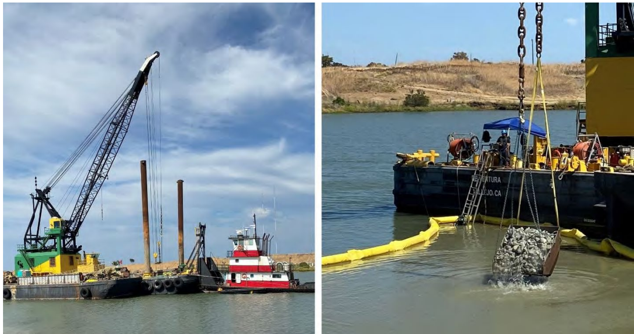
Figure 2-2. Photographs of a Derrick Barge Installing Rock
