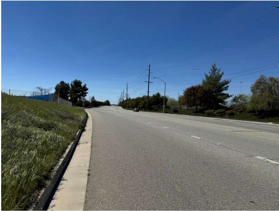
Exhibit 1.6. North driveway looking left (west) – 300-ft sight distance achieved
