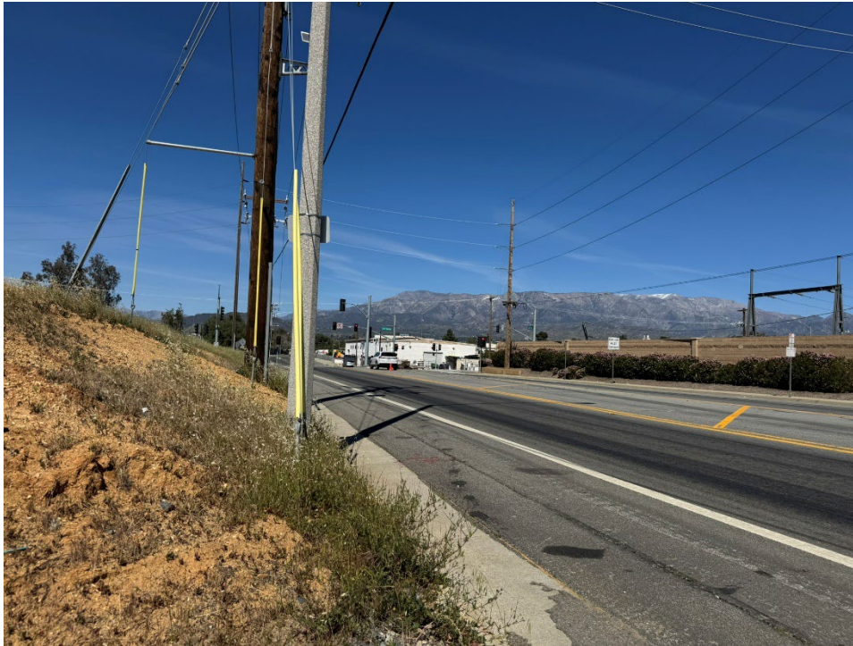
Exhibit 1.7. East driveway looking left (north) – 250-ft sight distance achieved after pulling forward
