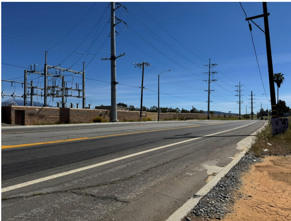
Exhibit 1.8. East driveway looking right (south) – 250-ft sight distance achieved
