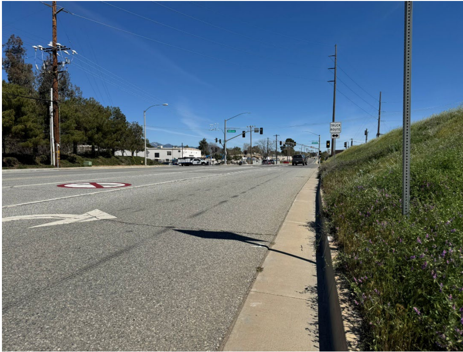
Exhibit 2.1. North driveway looking right (east); note solid white line and truck restriction pavement markings
