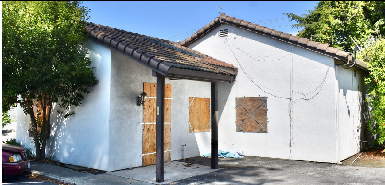
West façade, looking northeast
