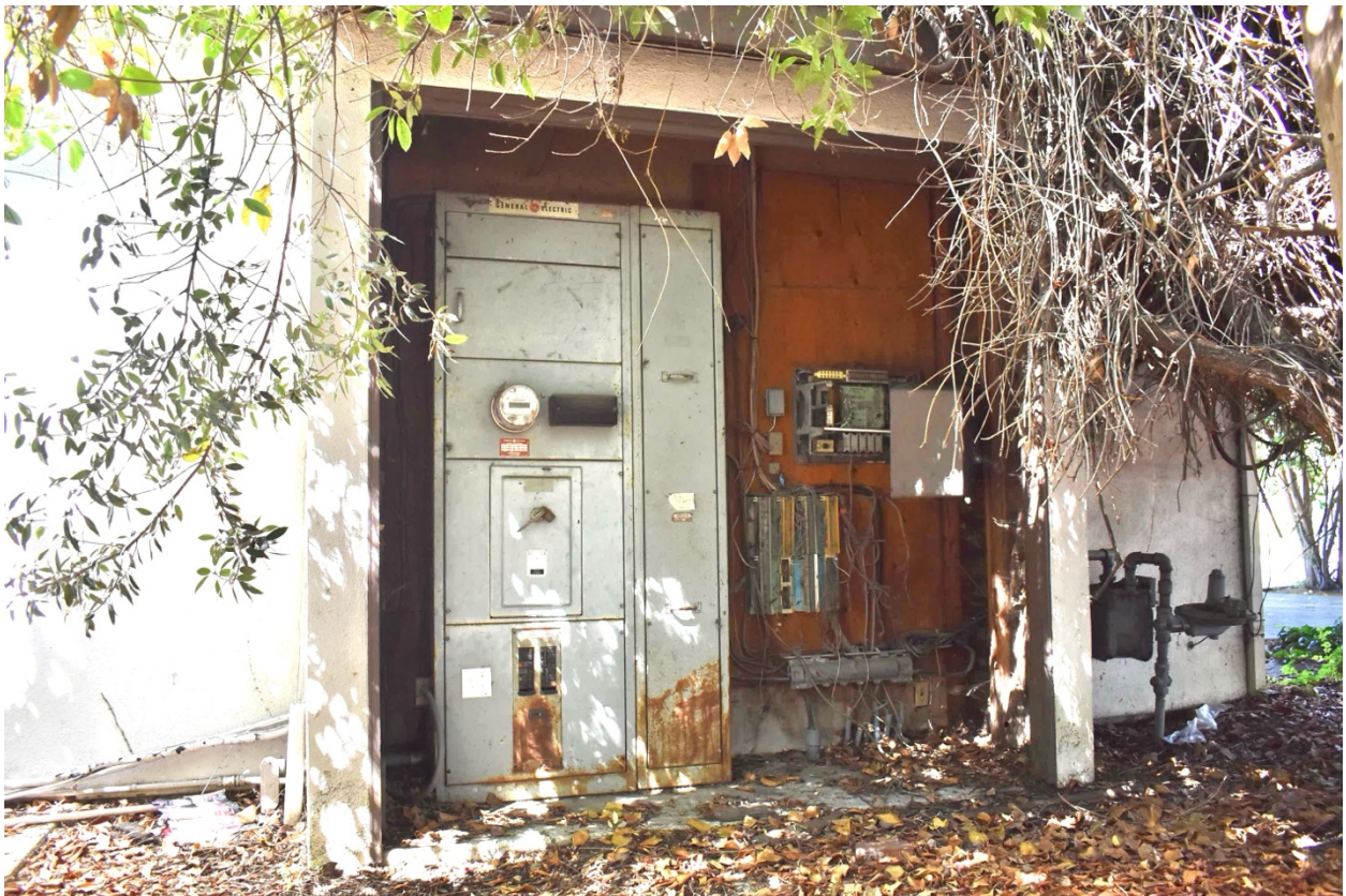
Utility shed on south façade
