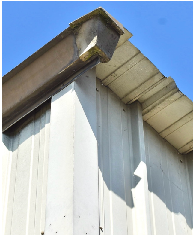
South façade (left); Roof detail (right)
