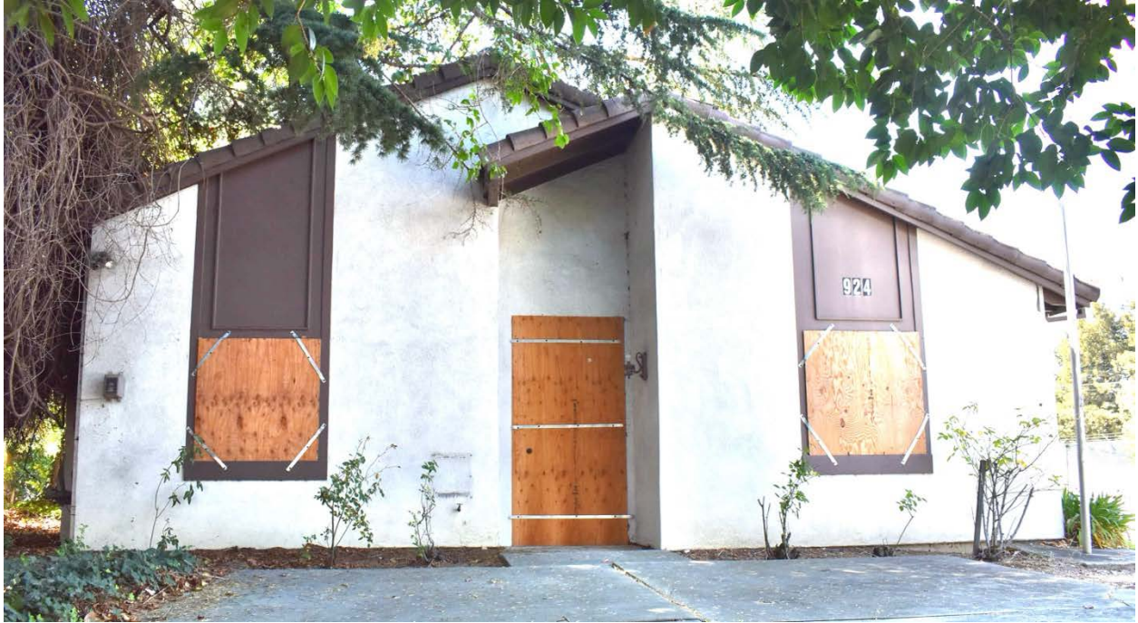
Figure 5: East façade (front entrance)
