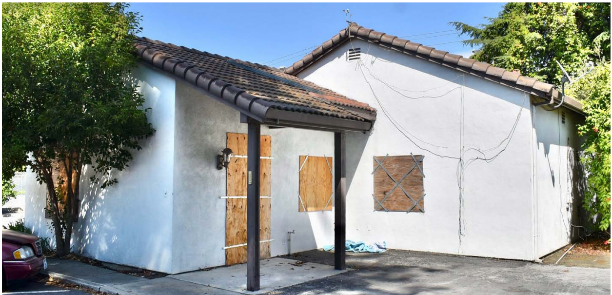
Figure 8: West façade, looking northeast
