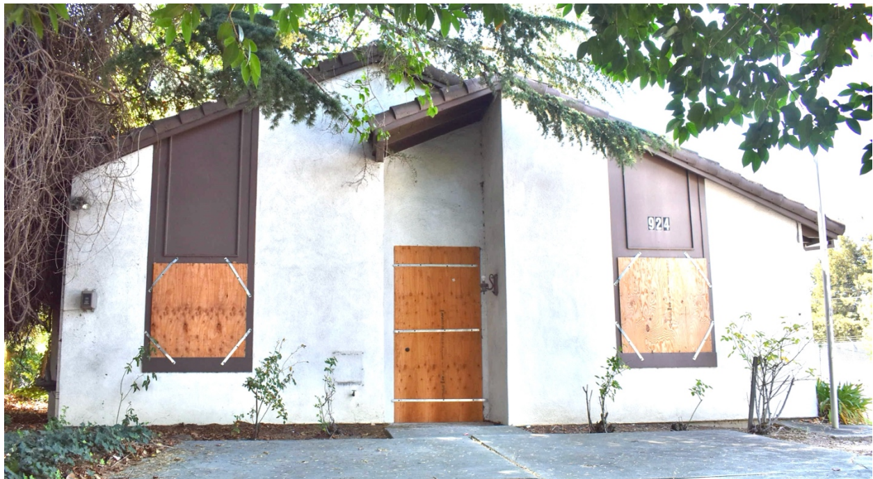
East façade (front entrance)
