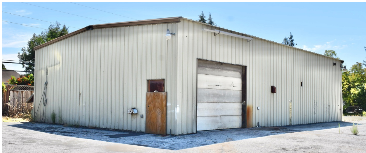
North and East façades, facing southwest
