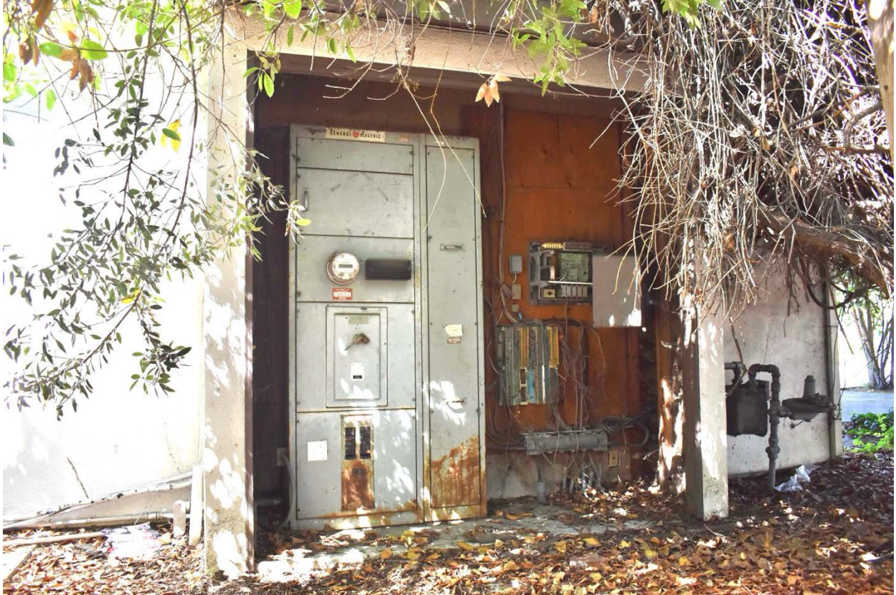
Figure 7: Utility shed on south façade
