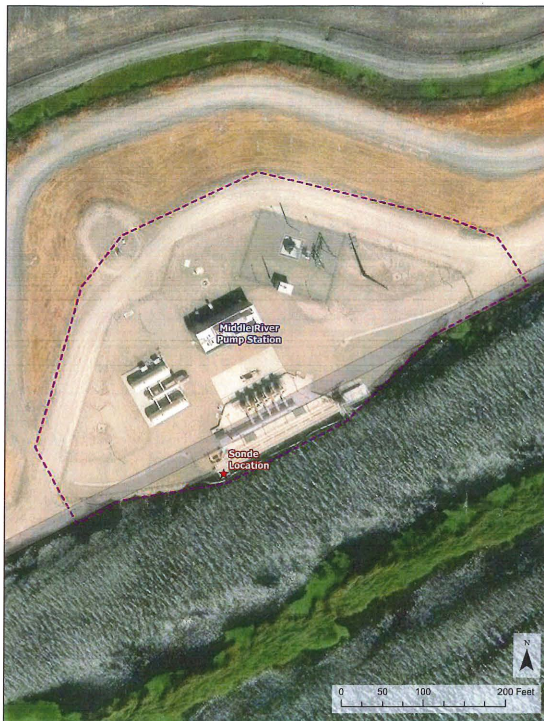
Figure 3: Middle River Pump Station Location Map
