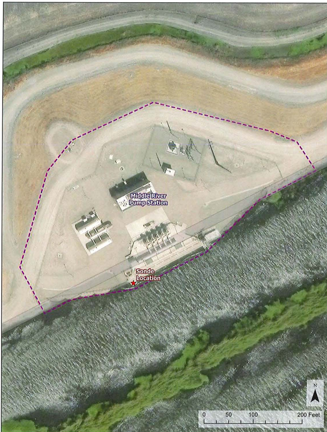
Figure 3: Middle River Pump Station Location Map
