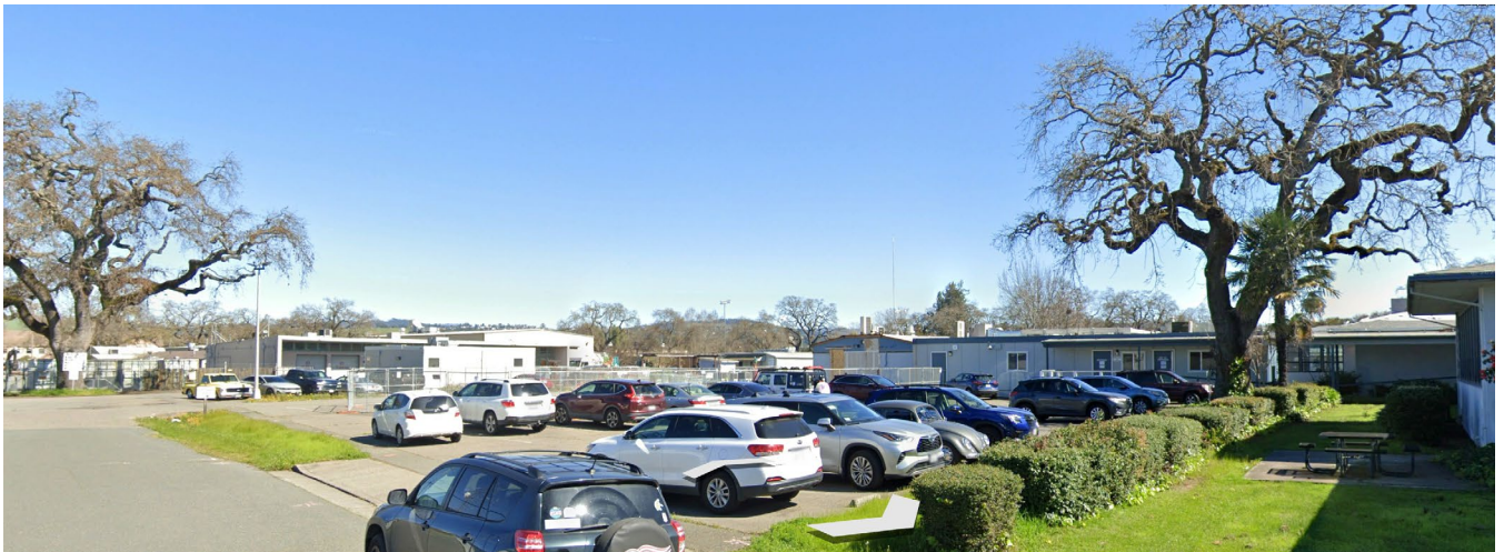
Facing northeast on Ripley Street with a view of the back of administration building (right) and maintenance facilities (background) and two Valley Oak Tree that would be protected in place.
