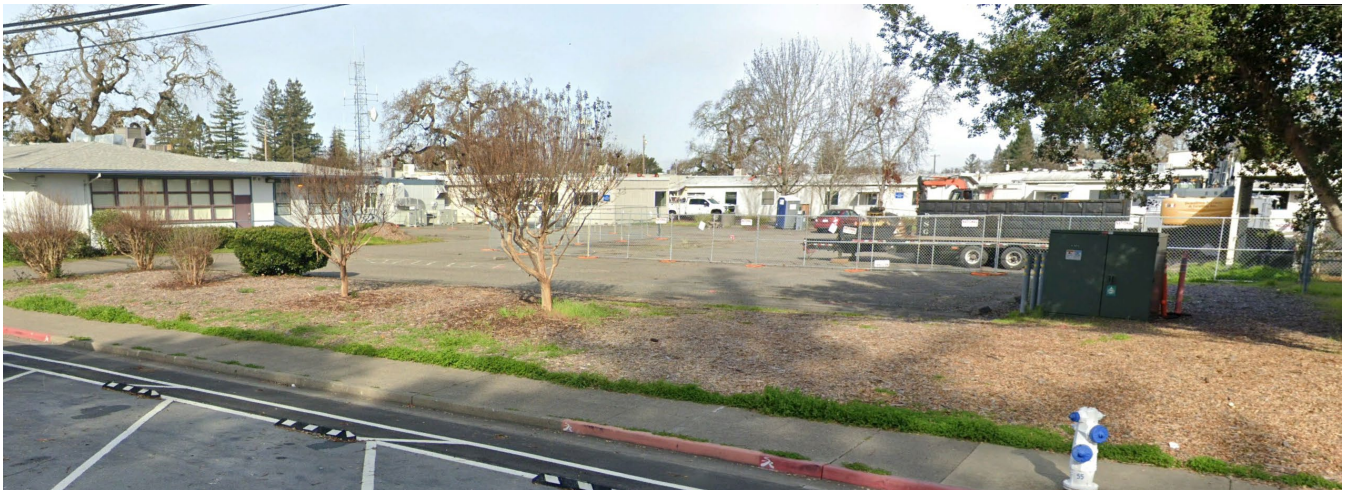
Facing northwest on Ridgway Avenue near southeast corner of Project Site.
