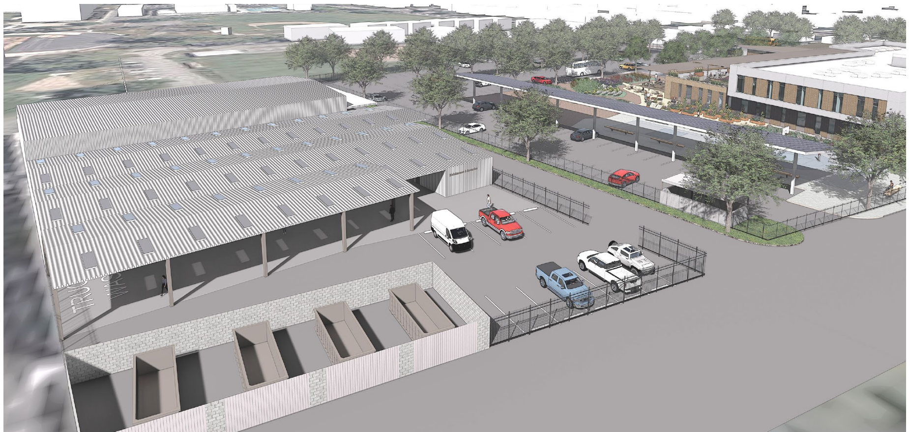
View of the M&O Facility with parking lot and truck wash.
