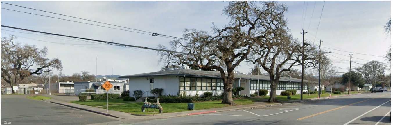
Facing northeast at the Ripley Street and Ridgway Avenue intersection with a view of the existing administration building and two Valley Oak Trees on Ridgway Avenue that would be protected.
