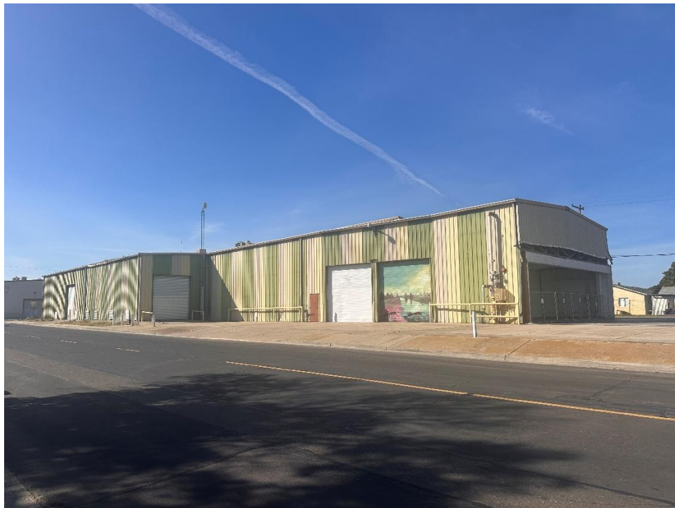
View of existing warehouse building at 641 Sixth Street, looking north
