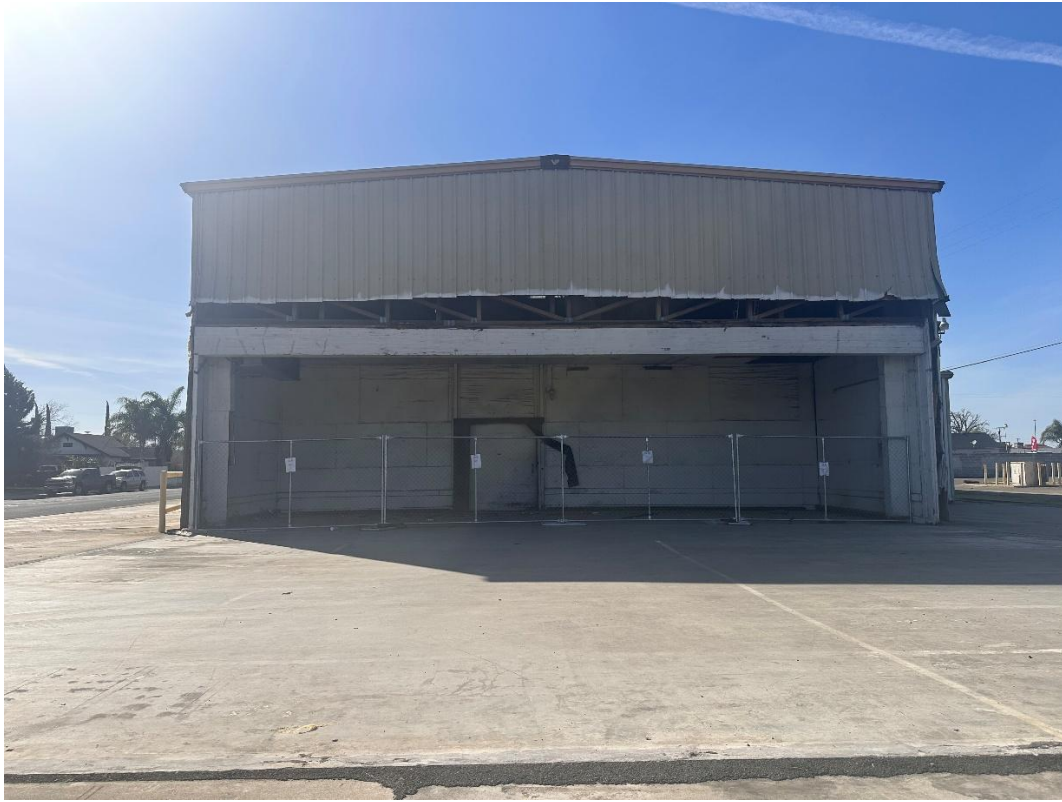
View of existing warehouse building at 641 Sixth Street, looking west
