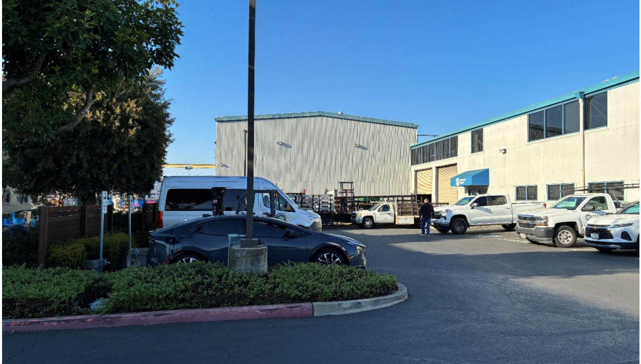
Photograph 3. View of the western façade of the existing main building, looking north from the site interior.
