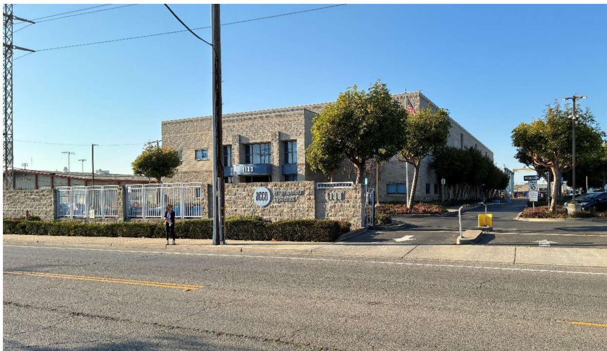
Photograph 1. View of project site frontage at the westernmost driveway on Aladdin Avenue and the southern façade of the existing office building to be demolished, looking northwest from across Aladdin Avenue.
