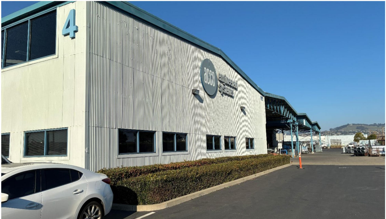
Photograph 4. View of the southern façade and canopy area of the existing main building, looking northeast from the site interior.
