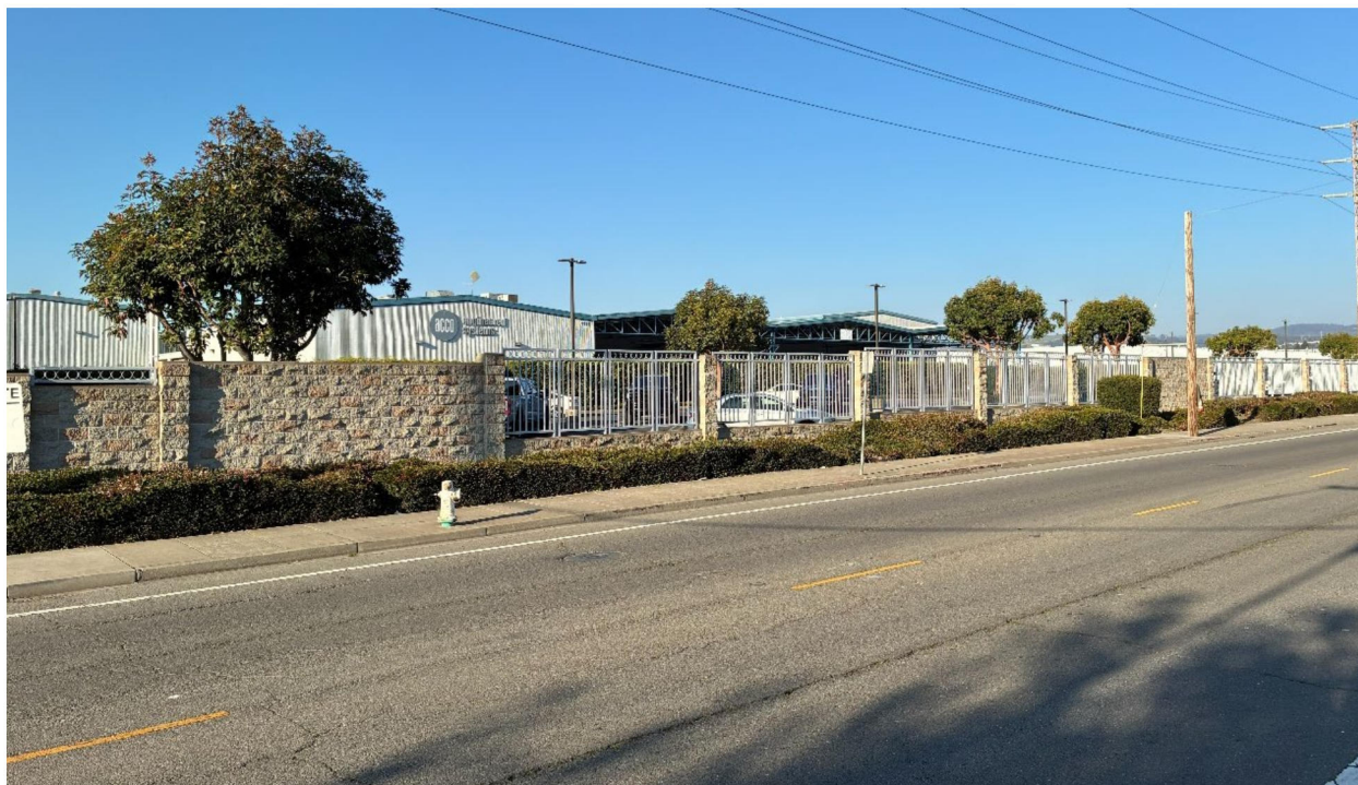
Photograph 2. View of project site frontage with southern façade of the main building, looking northeast from across Aladdin Avenue.
