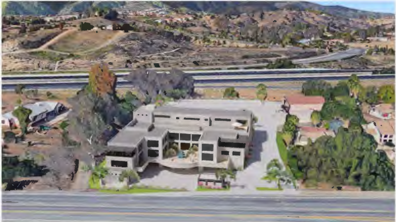
Figure 6B: Project Site Aerial View (After)
