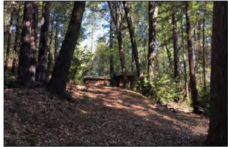
Existing cabins in the Study Area within the Douglas fir forest in the central portion of the Study Area
