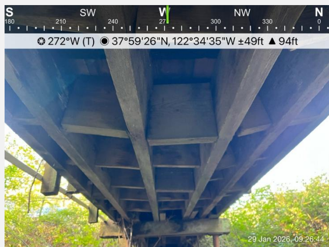
Photo 17. Underside of current pedestrian bridge where habitat was assessed for roosting bats.
