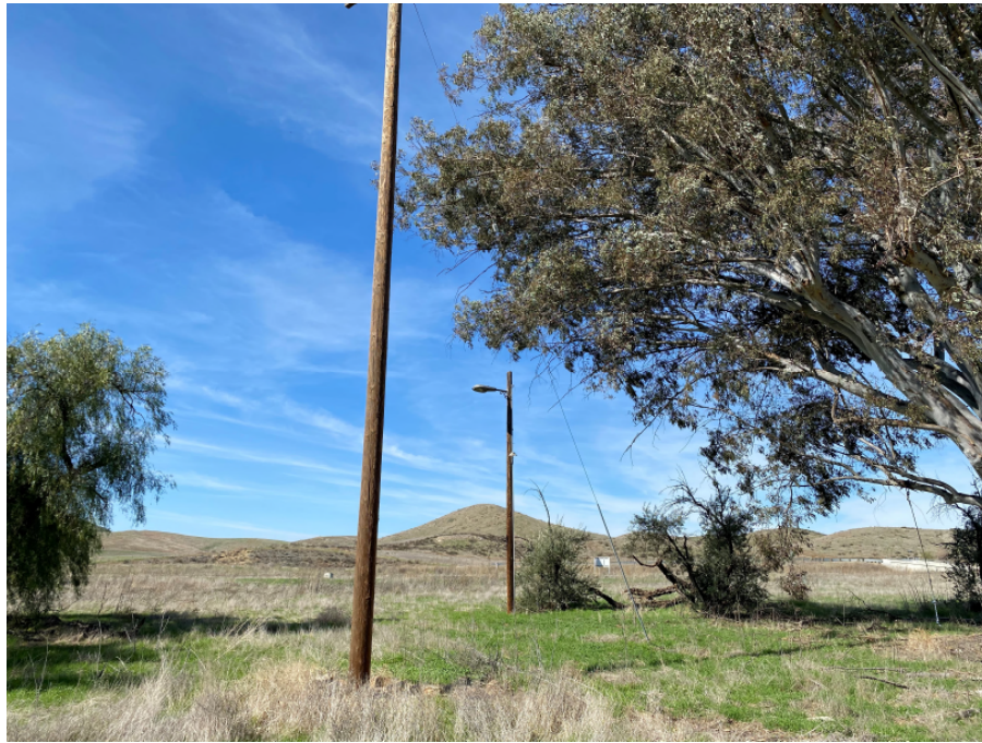
Photograph #11 Overhead power line and light post near the central portion of the Site.
