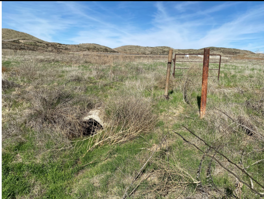
Photograph #15 Concrete drainage pipe located in the southwestern portion of the Site.
