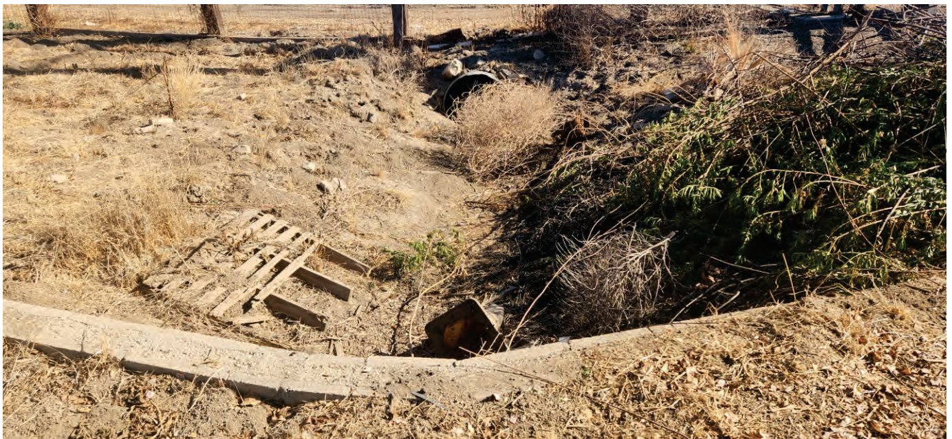
Photo 2: View facing east from Coventry Lane.
