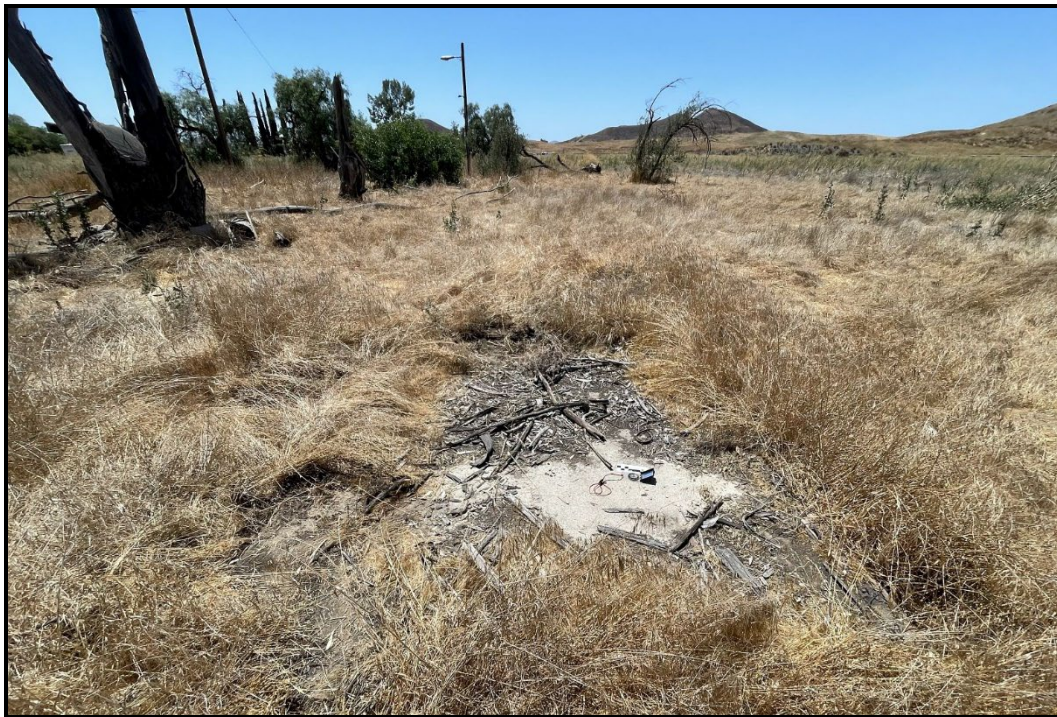
PHOTOGRAPH 17 Overview of Foundation 3 with Central Portion of Ranch Complex in Background, Looking West
