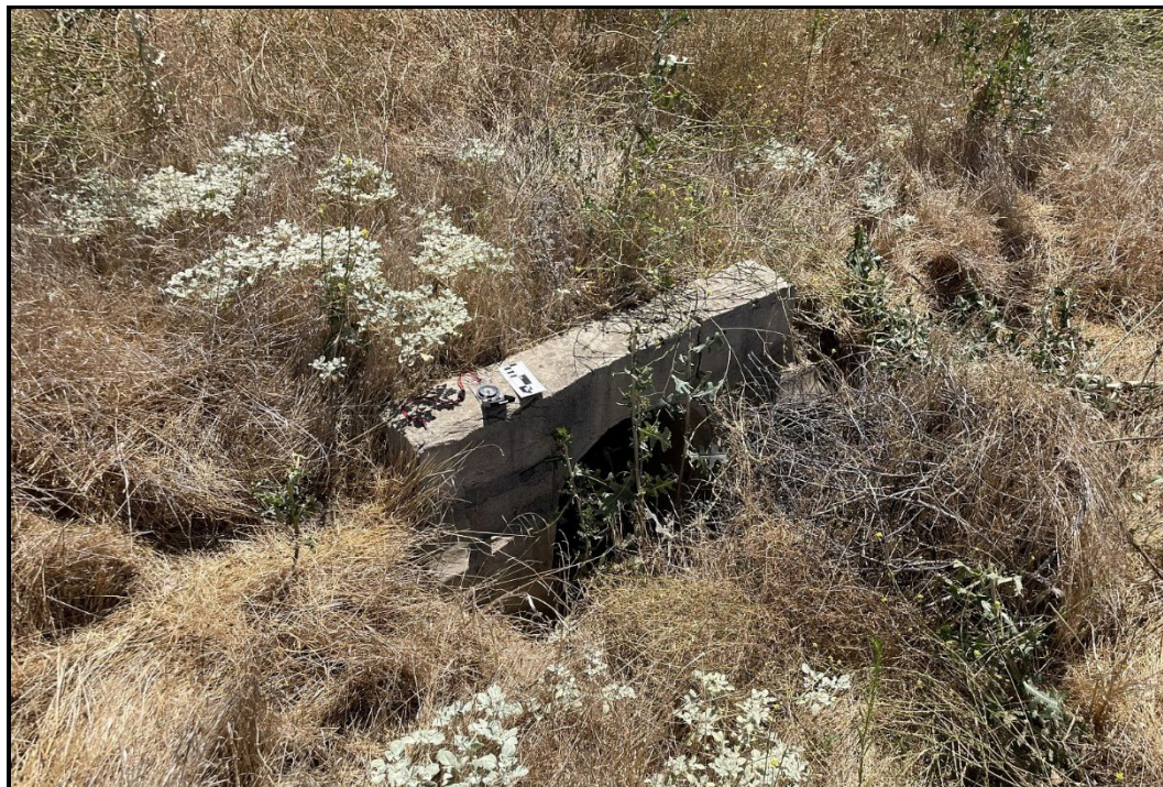
PHOTOGRAPH 18 Concrete Culvert Located on the North Side of Dilapidated Driveway, Looking Southwest
