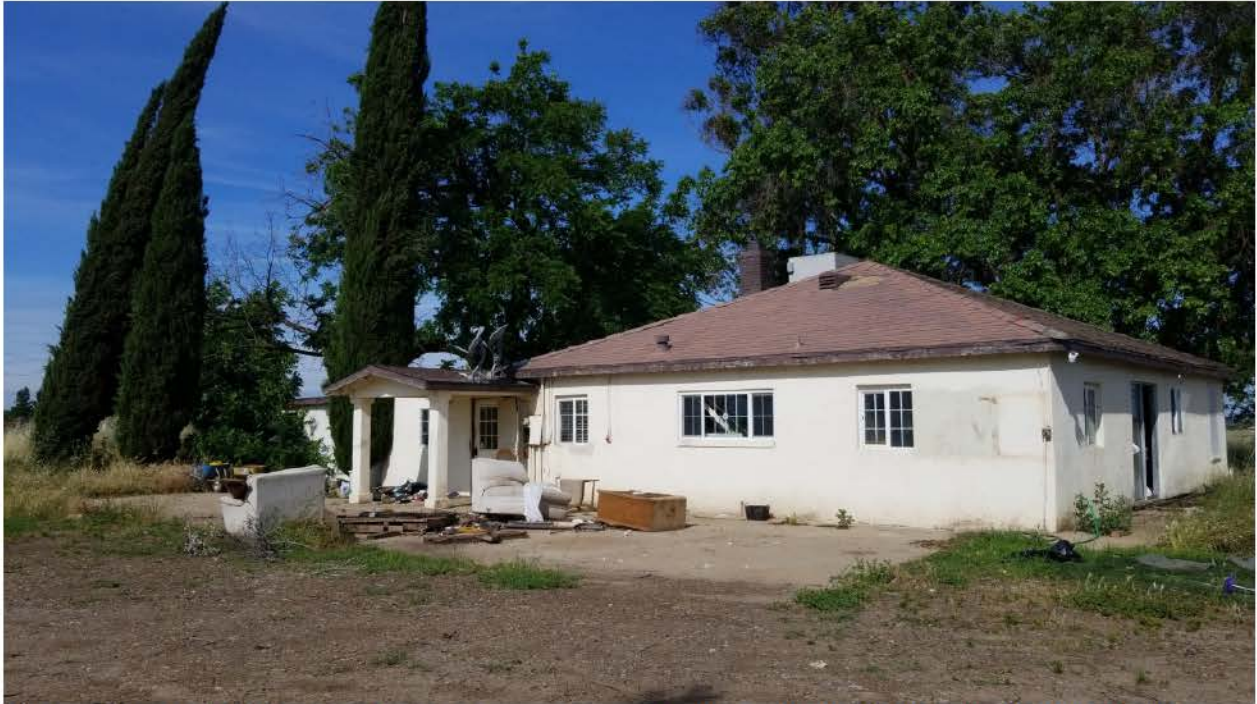
Photograph 1: Residence northeast corner, camera facing southwest, May 23, 2019 (AECOM).
