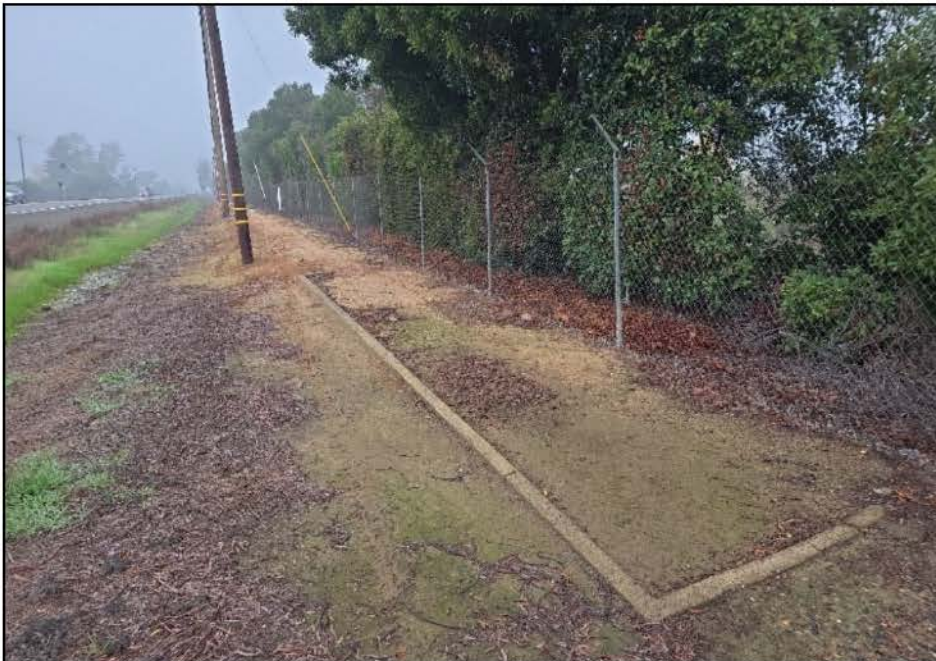
Photograph 12. Overview of Foundation 1 at P-34-005400, December 5, 2025.
