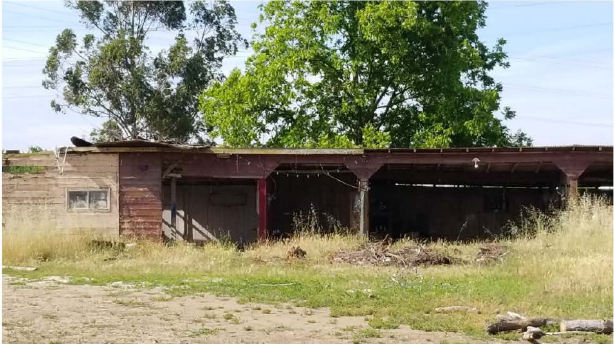
Photograph 3: Shed near residence with openings along north side, Camera facing south, May 23, 2019 (AECOM).
