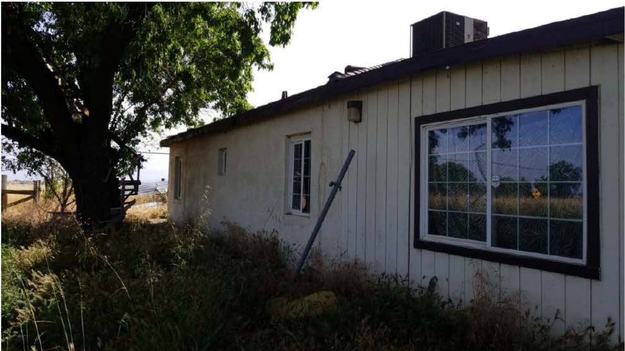
Photograph 2: Residence west side with rear addition, camera facing northeast, May 23, 2019 (AECOM).
