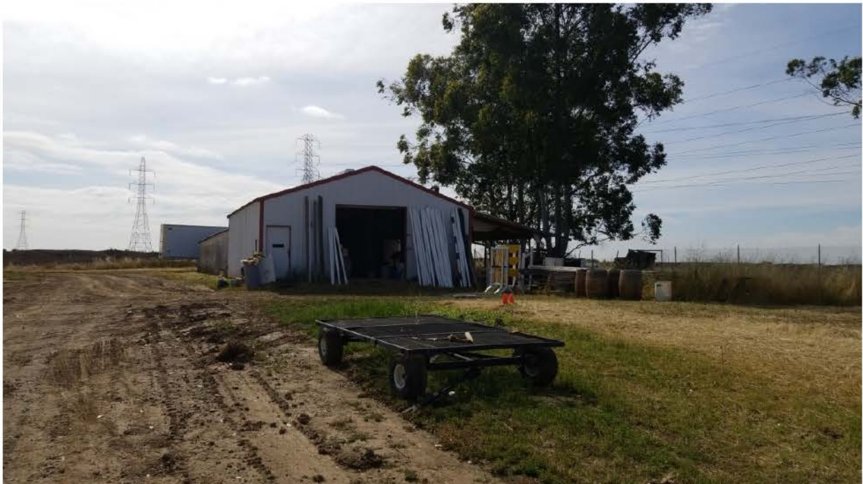
Photograph 4: West side of modern shed along east side of parcel, camera facing southeast, May 23, 2019 (AECOM).
