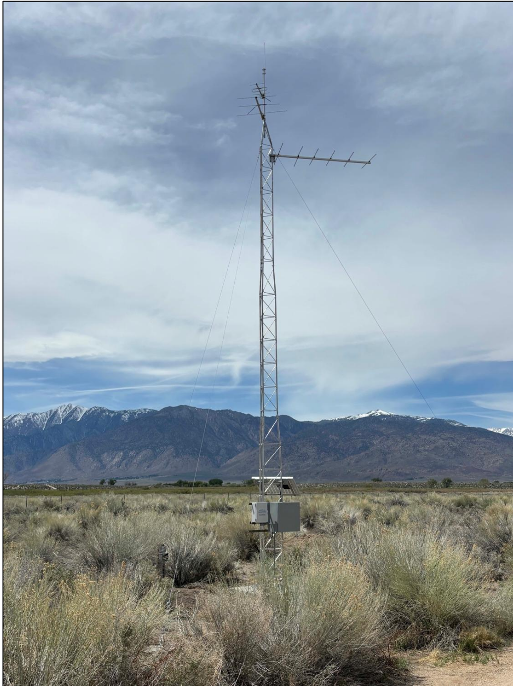
Figure 3. Example of a Motus tower already installed at a UC Nature research at UCLA's White Mountain Research Center. The proposed Motus tower at UCSB's SNARL would be nearly identical.
