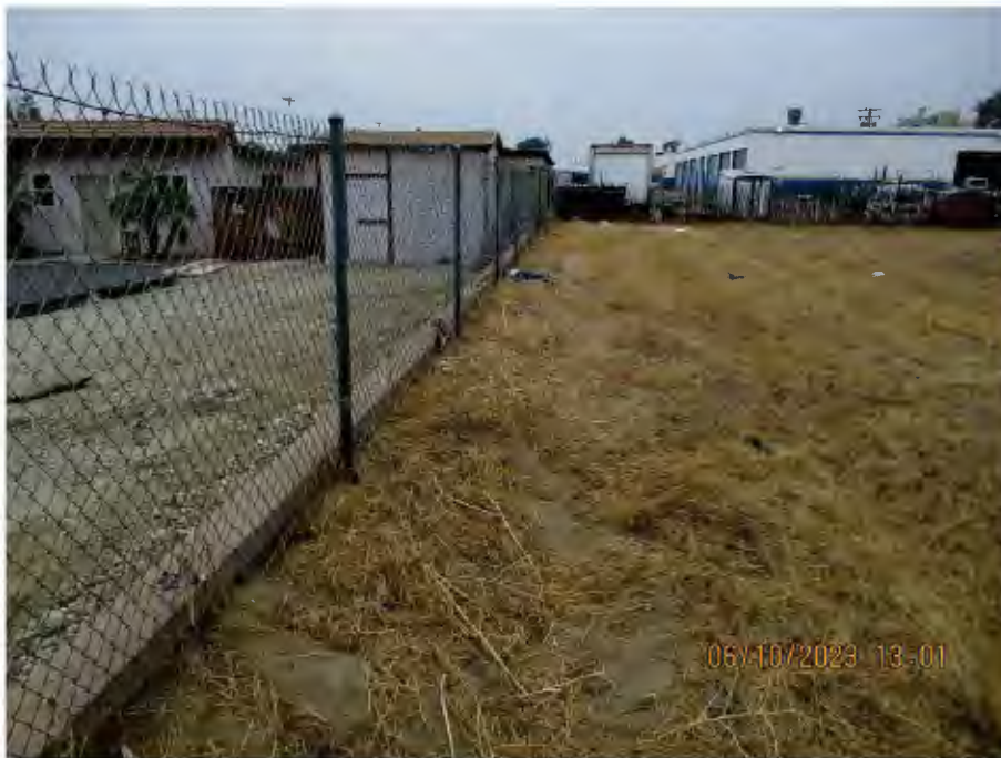
Photograph 4: Southwest project boundary – view north.
