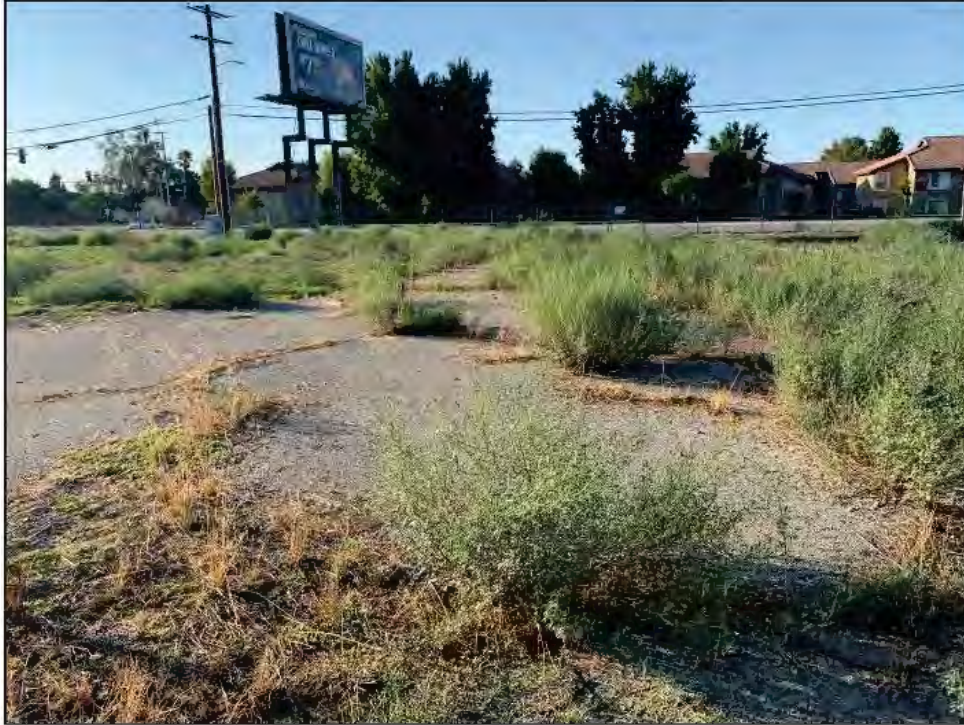
Photo 9. Asphalt Present in the Southern Portion of the Project Site, facing south.
