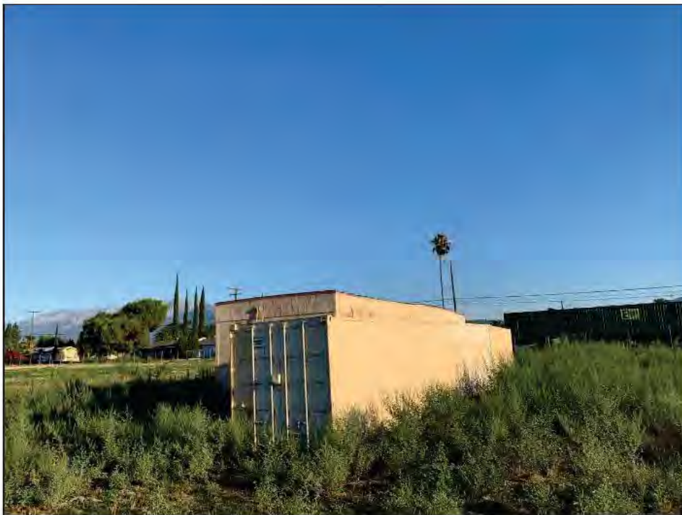
Photo 6. Portable Building and Shipping Containers near the North Side of the Project Site, facing northwest.
