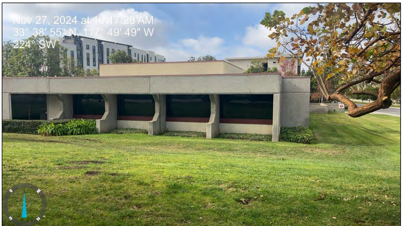
Looking southwest over the existing building found on Site A.
