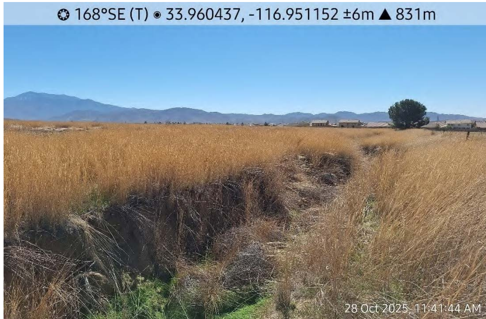
Photograph 5. View of drainage along western boundary of project site. View south.
