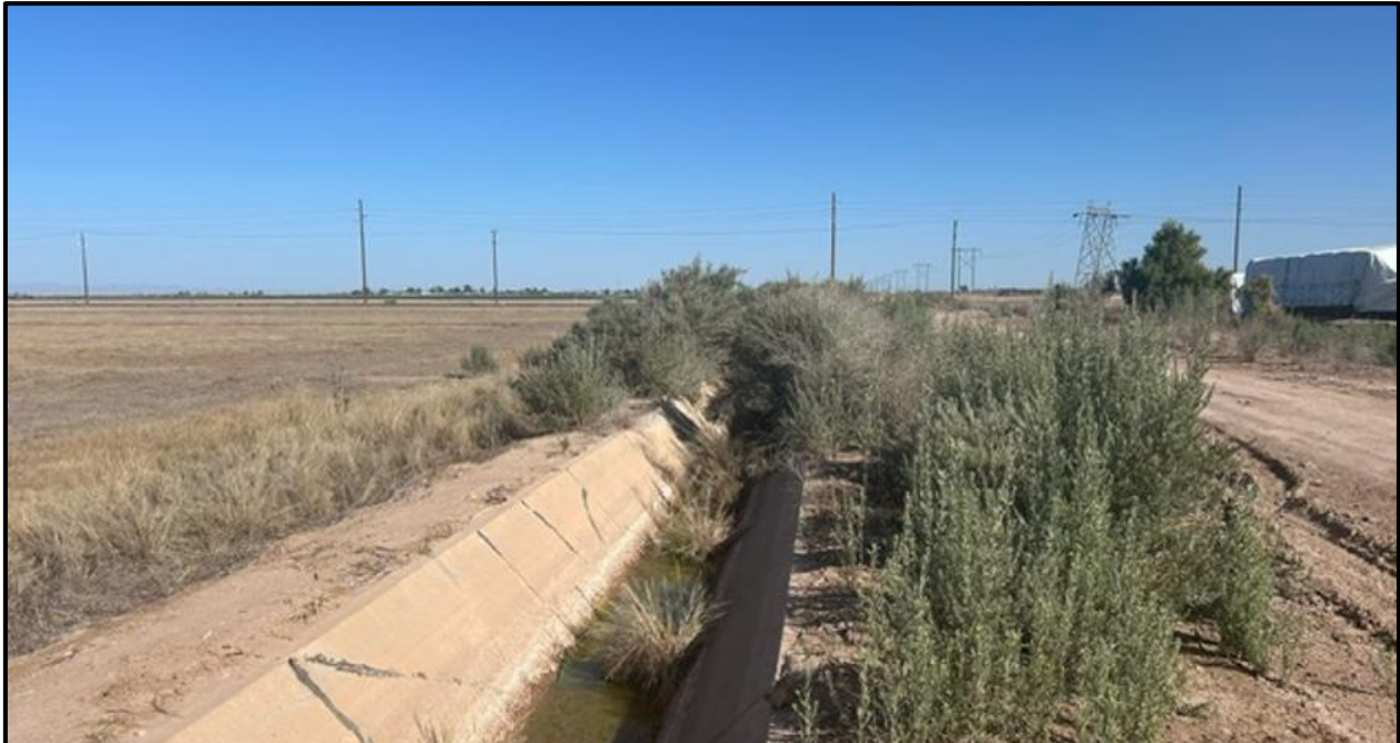
Photo 1: View from the just south of the Project boundary looking east along the concrete Stream Channel.
