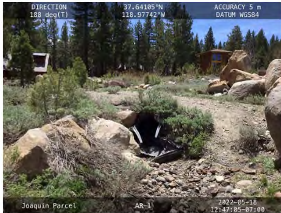
Photo 8. AR-1 at culvert crossing under graded dirt road. View looking south, upstream.
