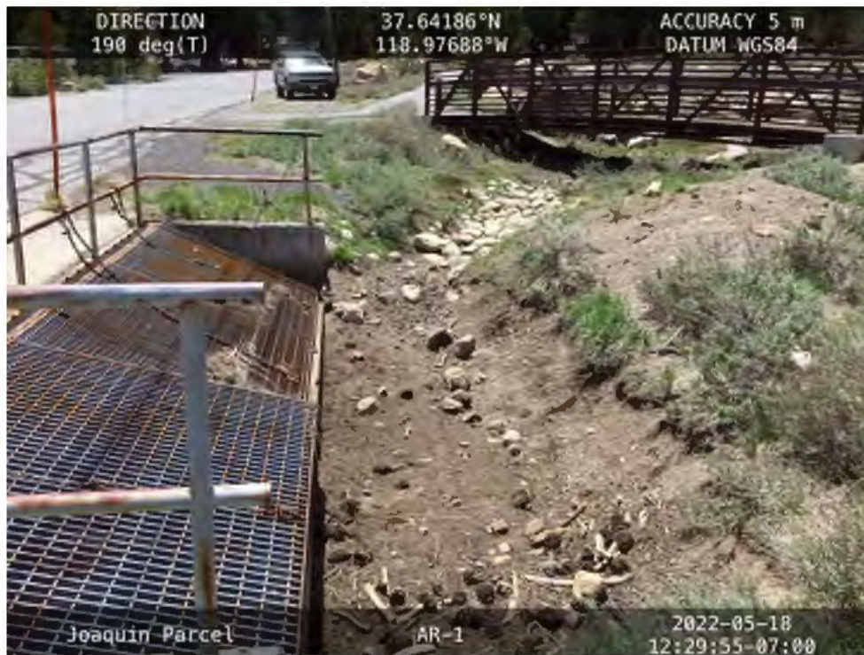
Photo 14. Location of where AR-1 exits the Survey Area through a grated culvert going under Joaquin Road. View looking south.
