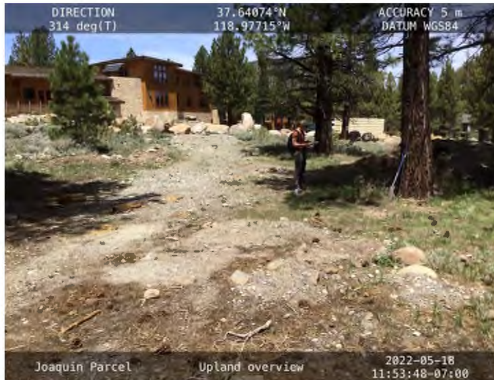
Photo 3. Overview of graded dirt road from east side of Survey Area toward AR-1 culvert crossing and leveled parking area on west side. View looking northwest.
