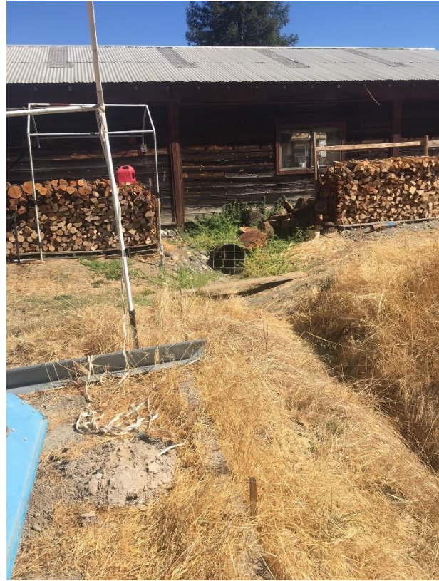
Culvert under barn
